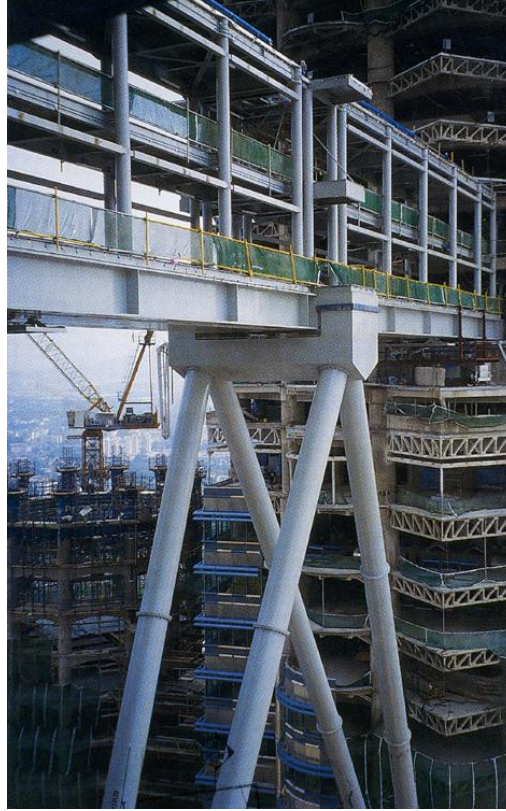
Şekil 5.4. 2 katlı Gökköprü (THE STRUCTURAL DESIGN OF TALL BUILDINGS, Vol. 6, 245-262 - 1997).
