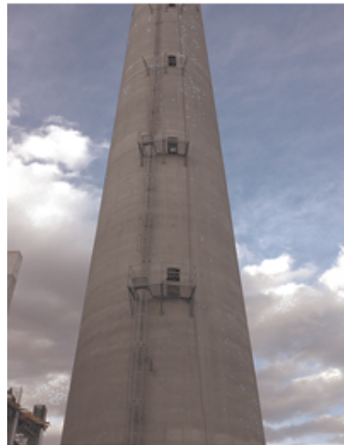
Figure 2.1. View of the Chimney at a Glass Factory Located in Bozuyuk.
