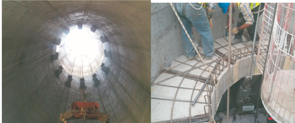
Figure 2.4. Precast Slabs and Corbels.
