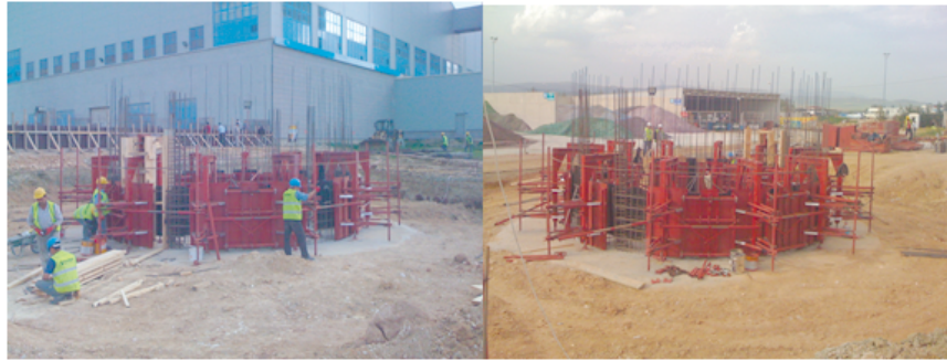
Figure 1.7. Setup Slipforming (ENDEM Co.).
