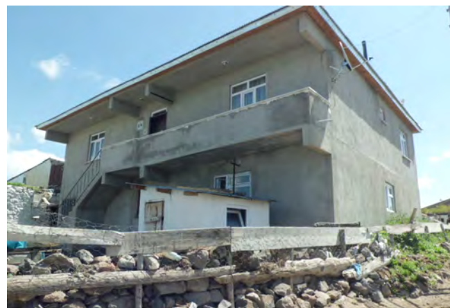
A view from a two-storey house built as RC frame structure.
