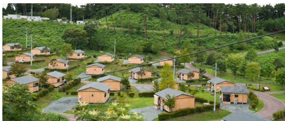
Figure 2.28 Transitional shelters built with timber composite (Sugawara and Hayada, 2012).
