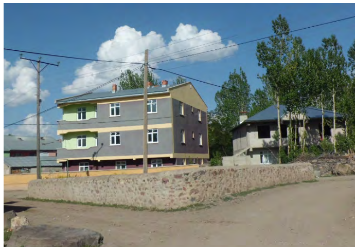
A view from a three-storey RC frame building.
