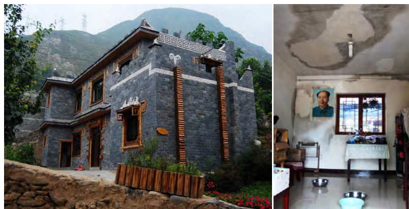
Figure 2.20 View of a Qiang house built in Pingtuo village (Aba Maoxian Department of Tourism, 2010) and the damp inside (Sheng, 2014).
