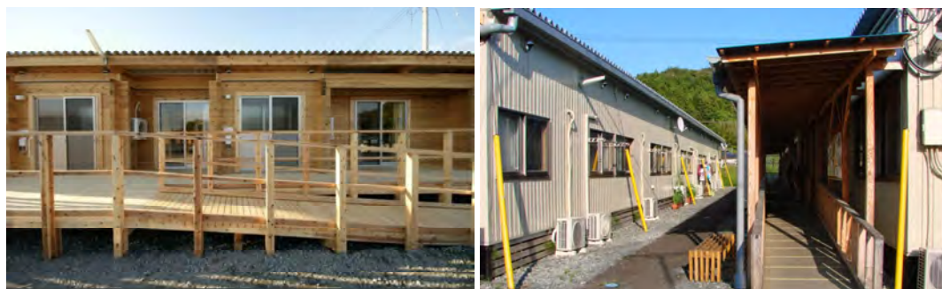
Figure 2.27 View of timber log temporary shelters built for a village settlement (IRP, 2013); temporary shelters built from container units (Alexander, 2014),
