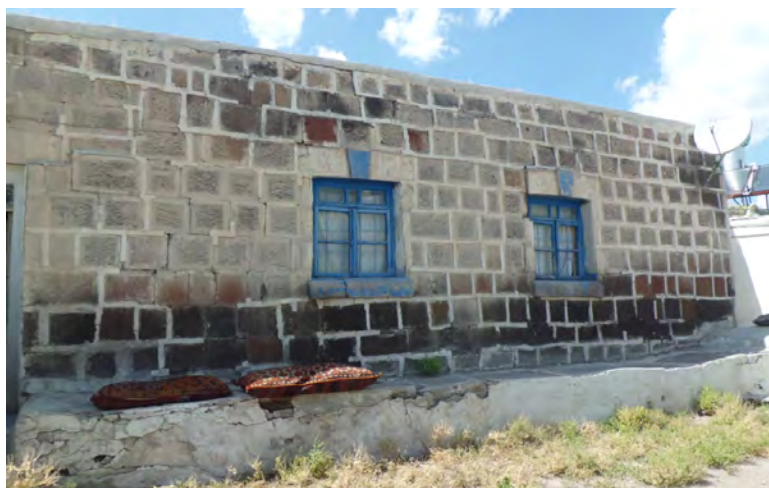
A view from a well-maintained stone masonry house, occupied.
