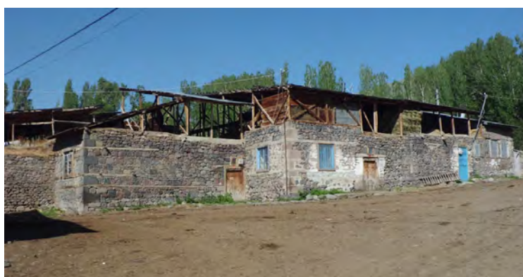
A traditional stone masonry unit including house, barn and storage.
