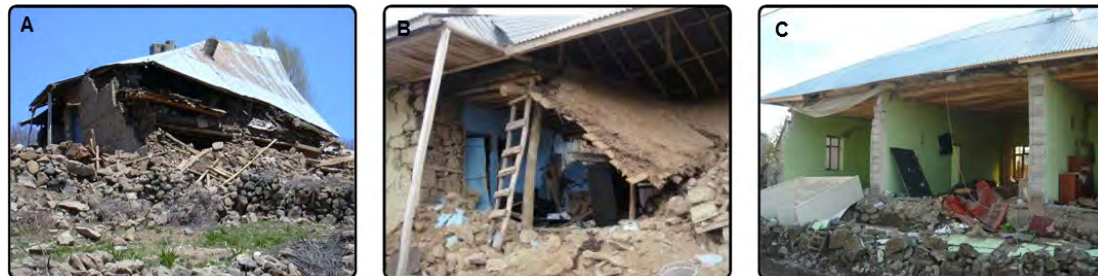
Figure 3.6 Examples of collapsed buildings from the earthquakes in Bingol, 2003 (A) (Karasin and Karaesmen, 2005); Elazig, 2010 (B) (Celeb et al., 2010); and Van, 2011 (C) (Kızılkant et al., 2011).
