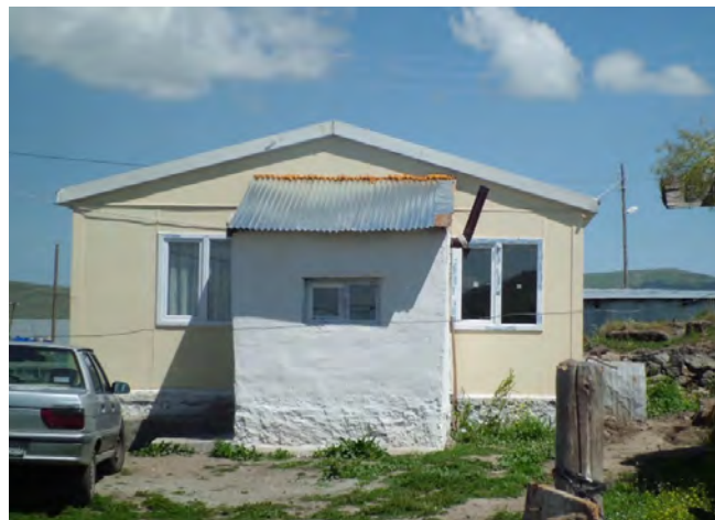
A view from a prefabricated house with an extension built with concrete blocks.
