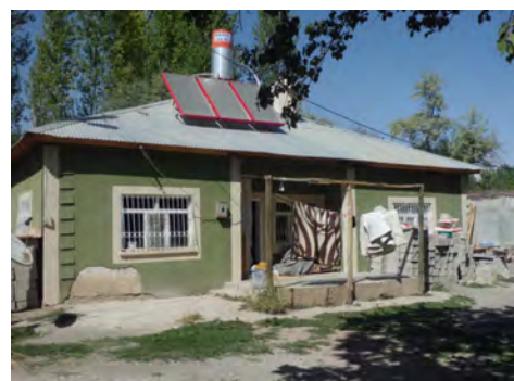
Figure 6 from top-down: the satellite map of Kasımoğlu; the abstract map shows the locations of the post-earthquake permanent houses built; a view from a permanent house under construction; and a view from the nearby former house still occupied by the same owner.
