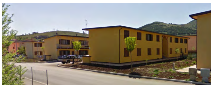
The two-storey blocks built in Monticchio village (Street view, May 2011, via Google Earth).
