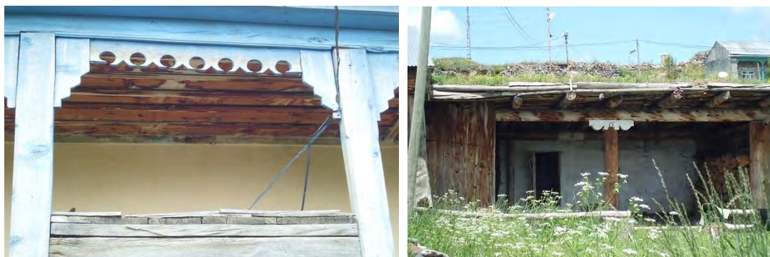
Figure 3.11: An example of the carvings on timber posts used in veranda and another example of a carving for the head of a larger timber post, which is an older structure.
