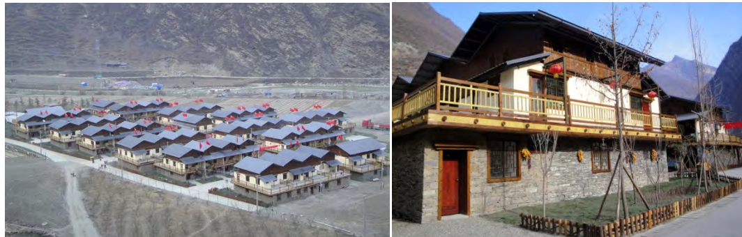
Figure 2.19 Settlement of Yang Liu village and a view of a house (Raskin, 2012; Archnet, 2010).
