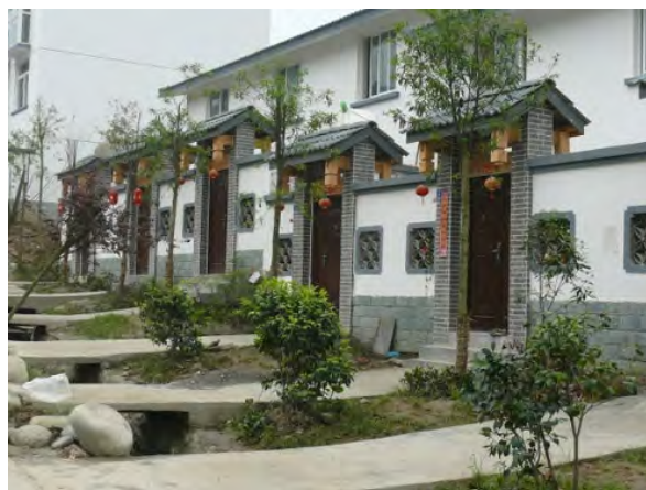
Figure 2.18: View from the entrances of houses built in Qipan village (50 Internet Media, 2009).
