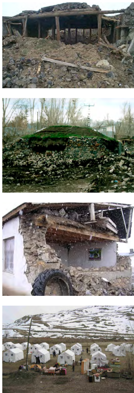
Figure 5.15 from top-down: a collapsed barn in the village of Alaca; a collapsed masonry house in the village of Tazegul; a collapsed house with very thick walls and heavy roof; and, a view from a tent settlement for temporary sheltering which is erected by the Turkish Red Crescent (Dogan et al., 2004; Korkmaz, 2007; Denizlioglu et al., n.d.; IFRC, 2004).
