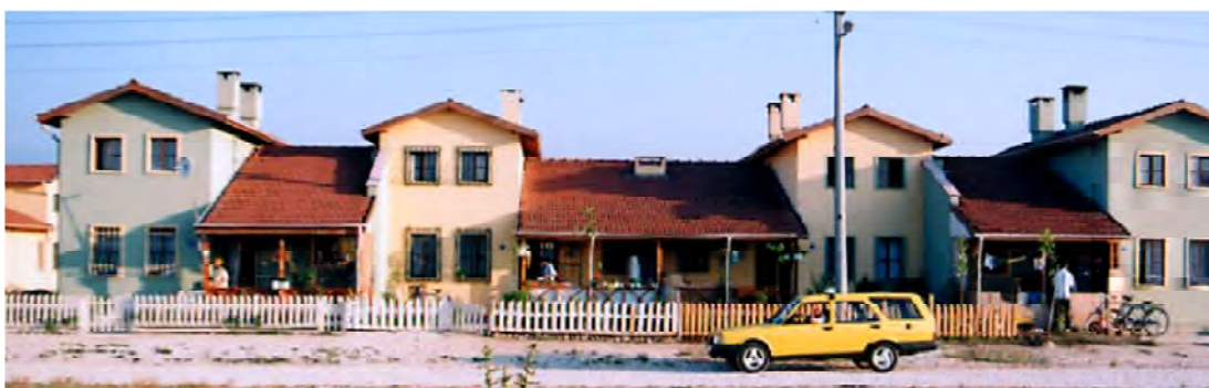
Figure 5.9 The view of the Beyciler social housing project in Duzce (Onder et al., 2010).
