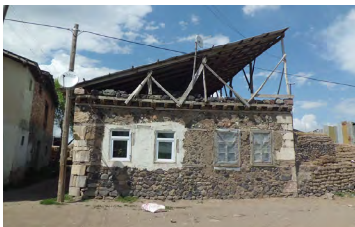
A view from a traditional house, the left hand side is residence and the right hand side is storage. On the roof, hay is stocked.
