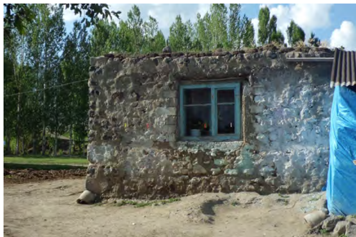
A view from a traditional masonry building occupied as a house.
