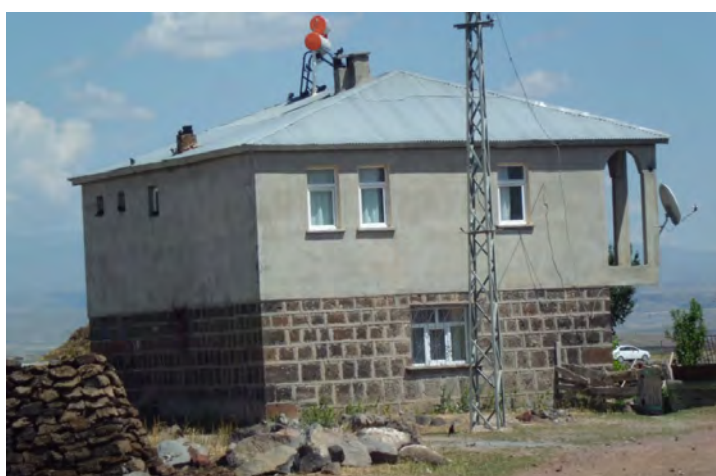
A view from a two-storey house, the ground floor is cut-stone masonry and the upper is RC frame with concrete block infill walls.
