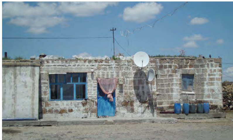
A view from a traditional masonry house built with cut stone.
