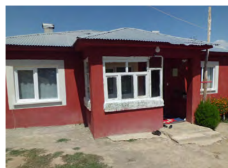
Figure 8 from the top-down: The view of the moderately damaged house that was still occupied by the owner; the barn unit transformed into a residential unit by the same owner; the extended terrace area both by closing the three-sided entrance and pouring concrete for further floor; and, another example of creating space from the entrance.
