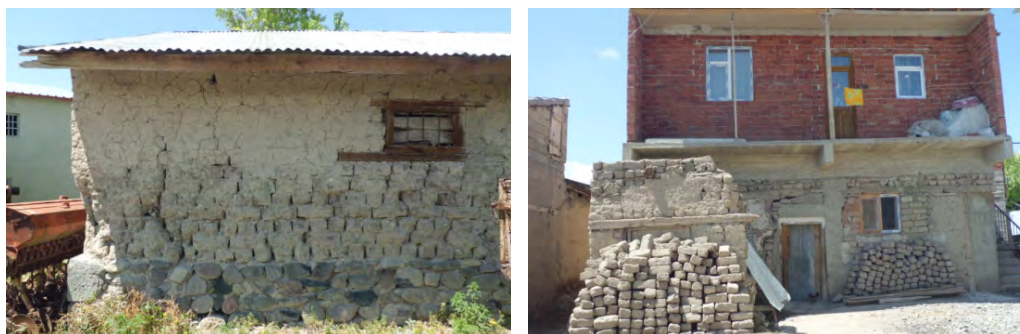
Figure 3.8 An example of adobe masonry barn and a house with an added upper floor on the ground floor with adobe brick masonry walls (Author).
