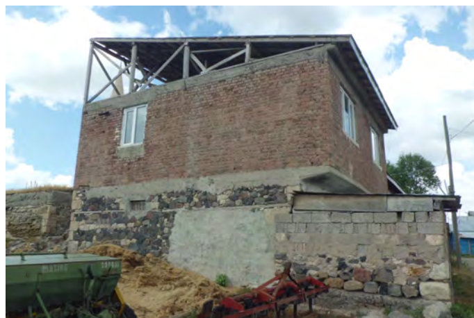
A view from a two-storey house, ground floor is stone masonry and the upper floor built on with poor RC ring beams with clay brick masonry walls.
