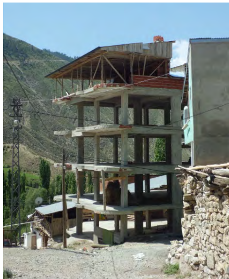
A multi-storey RC frame building under construction.
