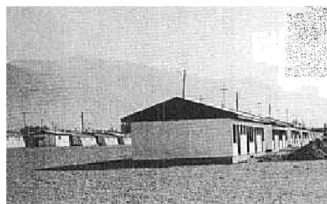
Figure 5.12 from the top-down: the units of the temporary hospital by the Turkish Red Crescent; the inside of the temporary hospital (Meguro & Nakano, 1993); and, the temporary prefabricated houses for the survivors (Celebi, 1993).
