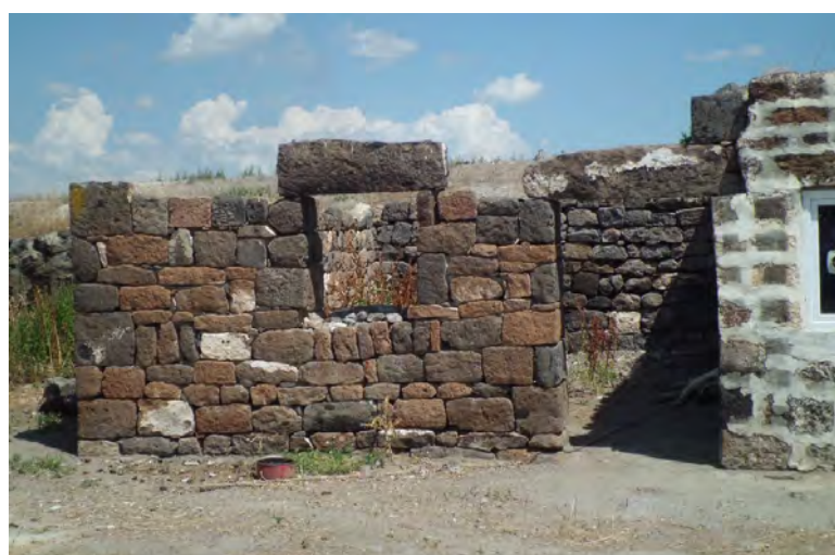
Ruins of a masonry structure built with shaped stone with no mortar.
