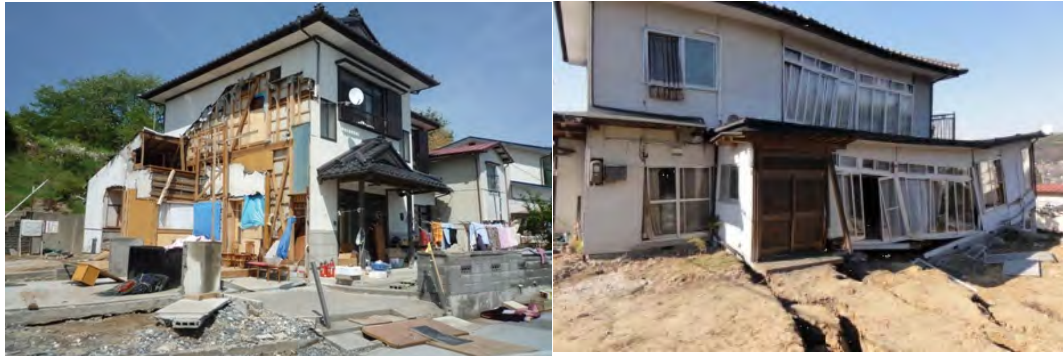
Figure 2.26 Wooden houses still standing but damaged by the tsunami (Koshihara et al., 2012); a residential building that suffered liquefaction (Hando and Fujita, 2011)
