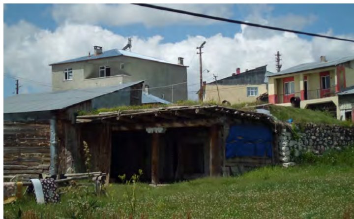
An overall view from the settlement, a traditional timber log-stone masonry storage in the front and newly built RC frame buildings at the back.
