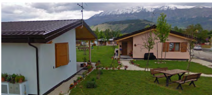
The M.AP project completed in Onna village (Street view, May 2011, via Google Earth).
