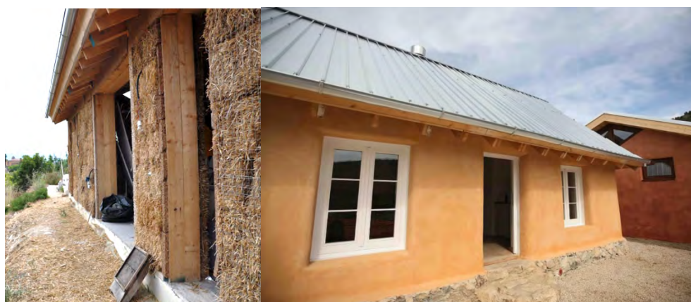
Figure 2.24 View of the straw infill in walls of a timber post-and-beam structure (Source: https://www.flickr.com/photos/41833955@N07/with/5062866349/ ) and a view of completed houses (Lisi, 2011).
