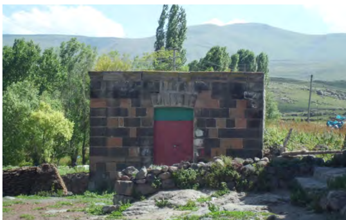
A view from a storage built with cut stone as masonry.
