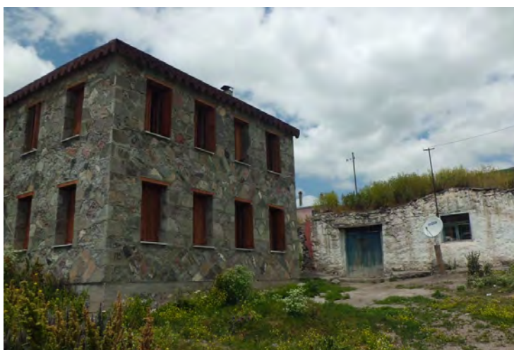
A view from a newly built two-storey stone masonry house strengthened with RC ring beams and cement mortar, and a traditional stone masonry house at the back.
