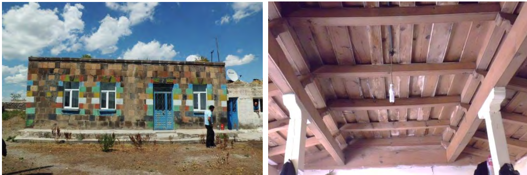
Figure 3.10 A villager's stone masonry house built with cut stone and a view of newly built timber post-and-beam roof.
