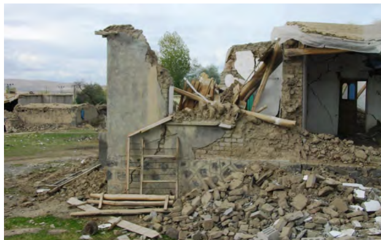
A collapsed adobe brick masonry house, Van, Turkey (EERI, 2012).
