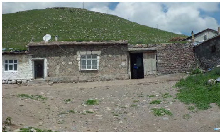
A maintained stone masonry house (with cement mortar) and its adjacent units.
