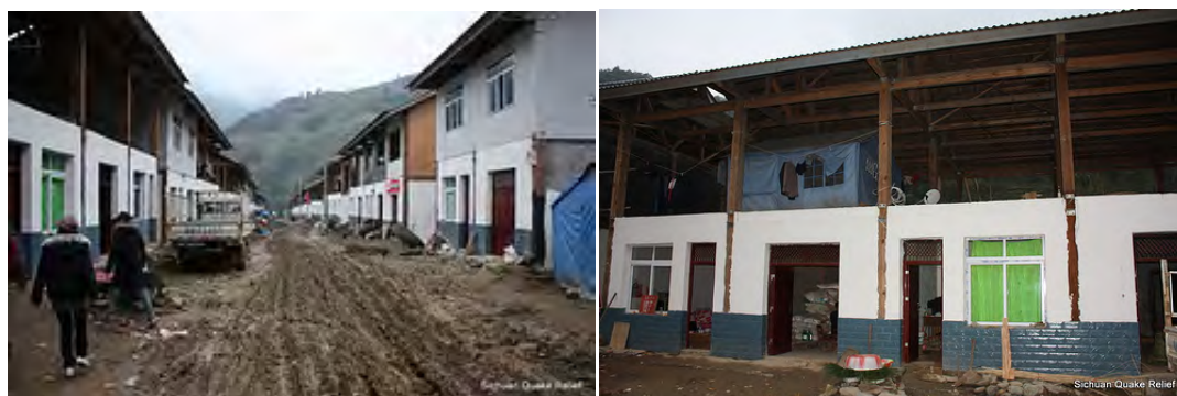
Figure 2.22 View from the village road of Yanyan and an example of a house under construction (Sichuan Quake Relief, 2009a).
