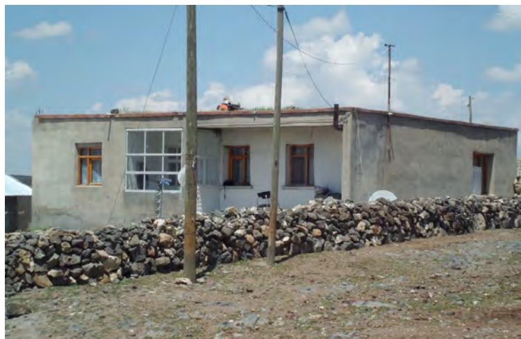
A view from a house plastered and extended with concrete.
