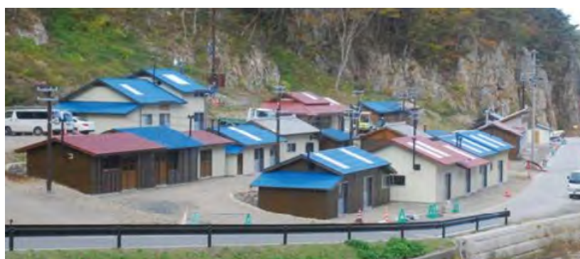
Figure 2.29 View of the permanent houses built in Tanohata (Foreign Press Center, 2014).
