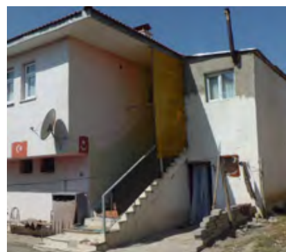
Figure 5 from the top-down: an example of a shed added to the entrance of a single storey house in the former settlement of Cigdemli; the general view of two-storey buildings built in the new settlement; a two-storey building with an added room next to the house; and the extension of the entrance of a two-storey house.
