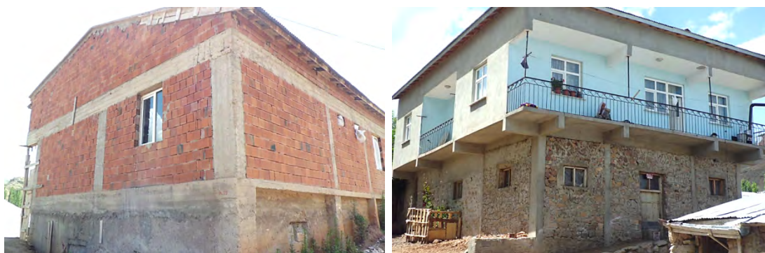
Figure 3.14 An example of RC frame structure with disproportionate and discontinuous columns and beams, and an example of a two-storey RC frame house with stone masonry infill ground walls.
