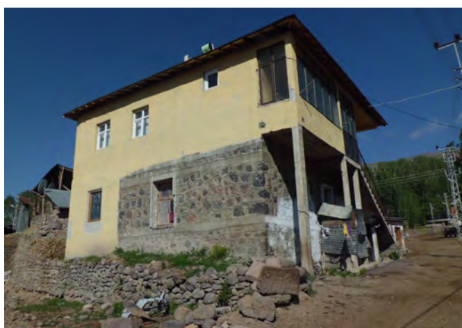
A view from a two-storey house built as extension from the stone masonry building in the ground floor.
