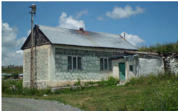
A view from a seasonally occupied stone masonry house with RC frame.
