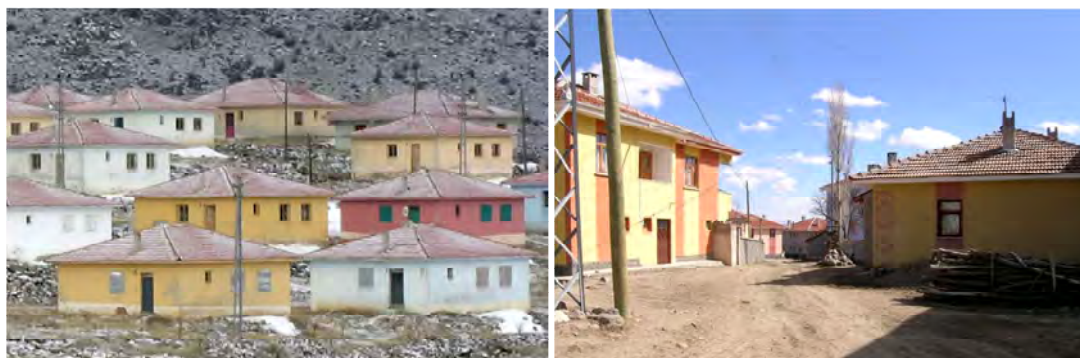
Figure 5.3 The unoccupied housing implementations in Çankırı, Elden village. on the left. The occupied implementations built in the existing location in Buguogen village (Dikmen, 2006).
