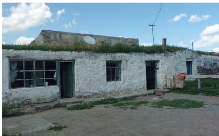
A view of another traditional stone masonry house and its nearby storage.
