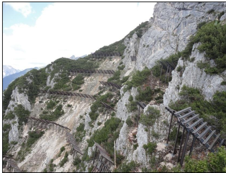
Figure 65. Snow bridges at the release zone (Photo: Kurt, 2011)
