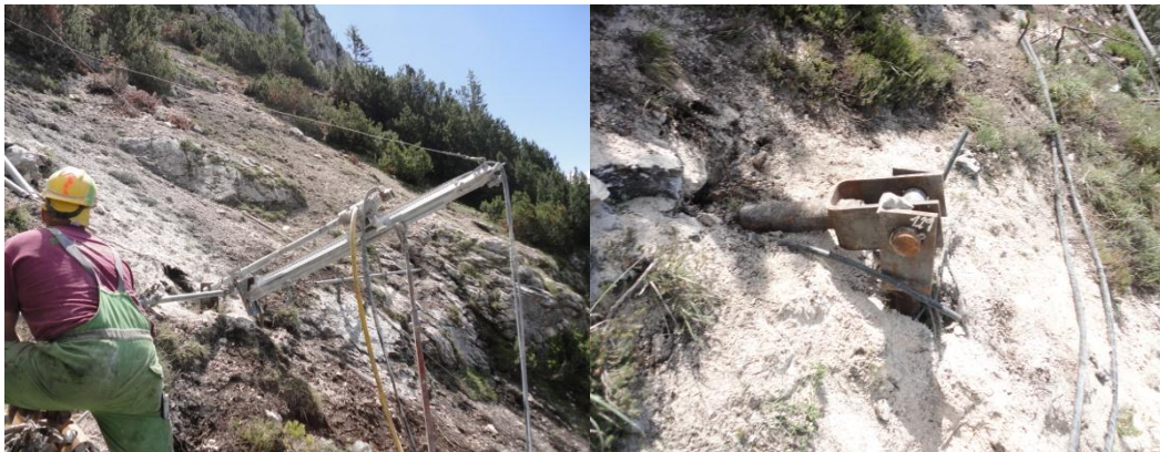
Figure 70. Compressive loading for an anchor (Photo: Kurt, 2011)
