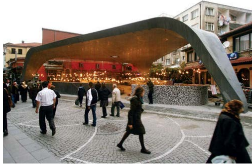
Figure 2.30 : The permanent Fish Bazaar canopy by GAD in Beşiktaş, İstanbul (URL-20).
