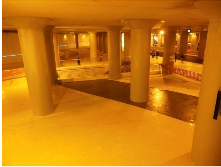
Figure 3.44 : Taksim Cumhuriyet street underpass photograph from entrance 1 showing bus stop area for Elmadağ destination and Taksim Subway line passage.
