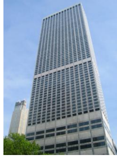
Şekil 2.19 Water Tower Place (Chicago) [44].
