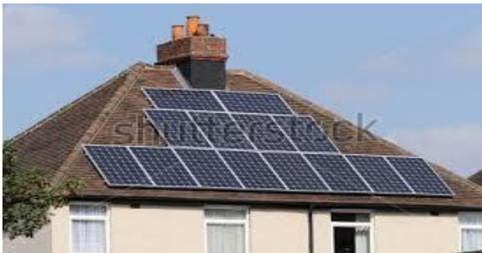
Figure 2.21. PV panels on a roof [29]
