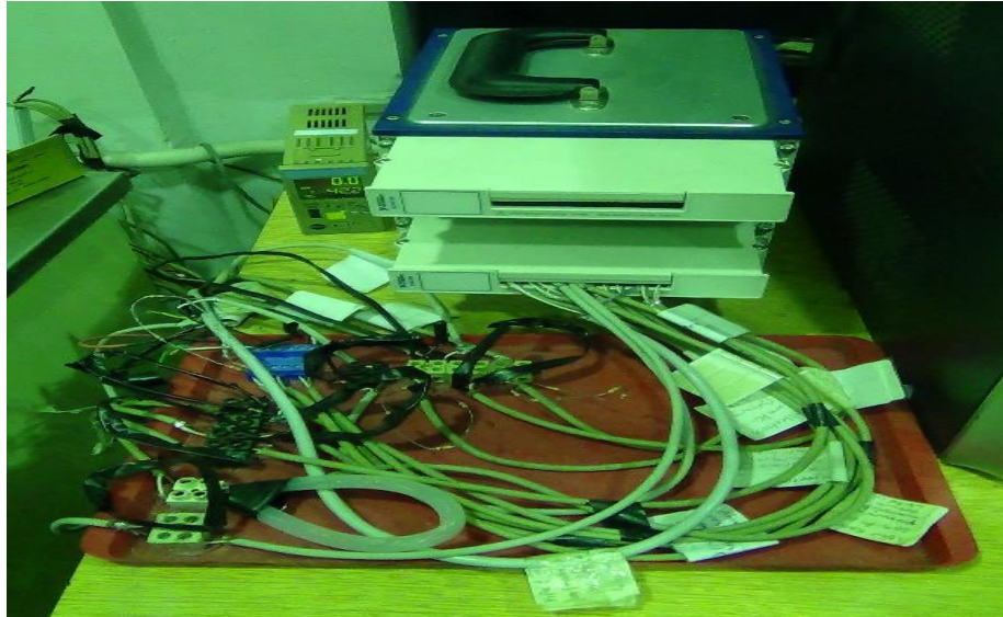
Figure 3. 16 Data logger and Acquisition System (National Instrument NI SCXI-100)
