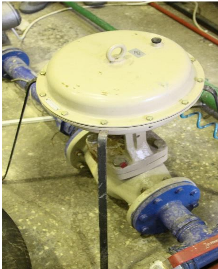
Figure 3. 11 Fisher Pneumatic Control Valve
