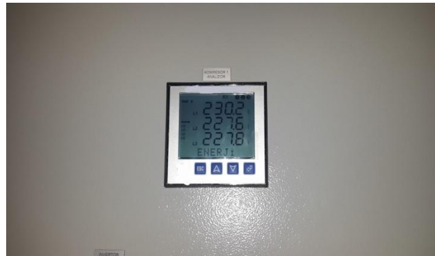
Figure 3.8 CO2 Compressor Energy Analyzer
