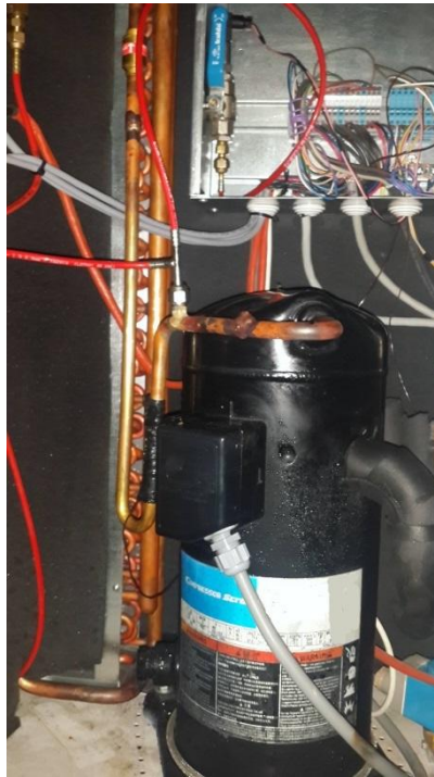
Figure 2.5 HTC Scroll Compressor and sensor connections
