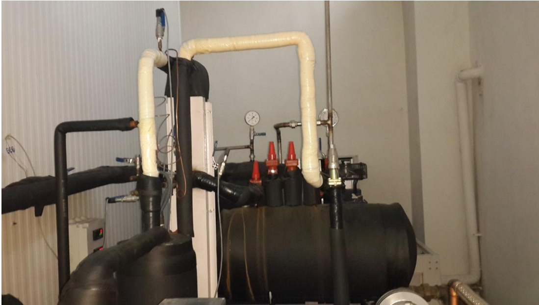
Figure 2.9 LTC PHE and Liquid Receiver
