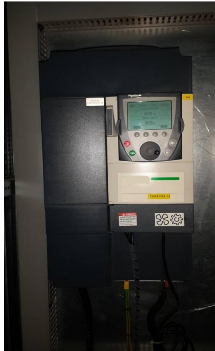
Figure 2.6 R404A Inverter placed on the Electrical Control Unit
