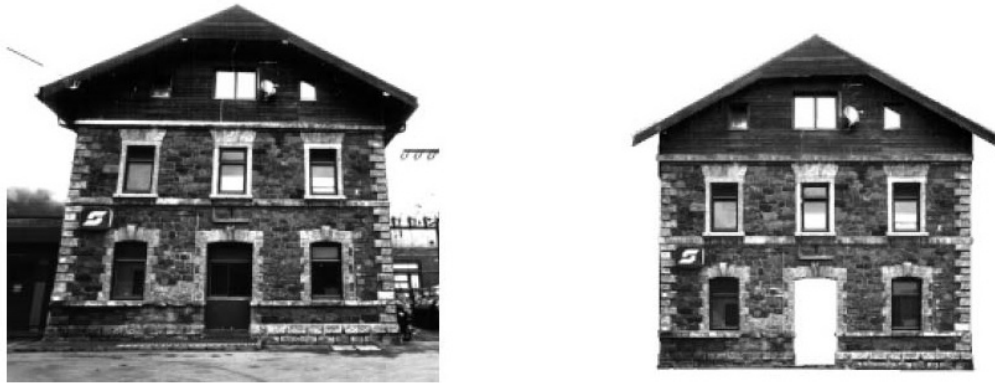
Figure 2.8 : Original and rectified (in scale) photographs of a façade.
