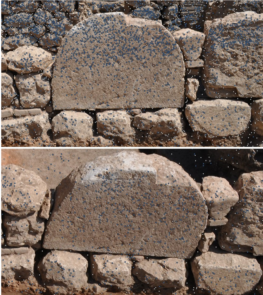
Figure 3.6 : Determined feature points on two overlapped images (blue ones were matched successfully while white ones couldn't be matched).
