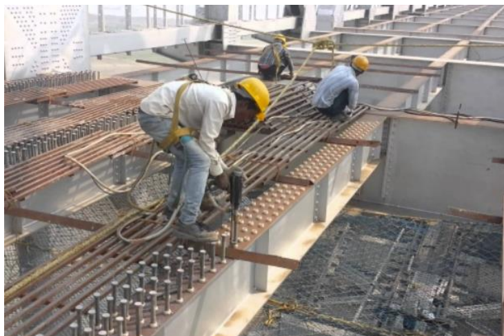
Figure 3.8 Instance of Arc Stud Welding Application in Boiler Manufacturing
