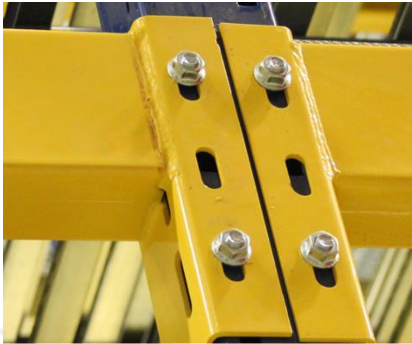
Figure 21. A typical bolted connection .
