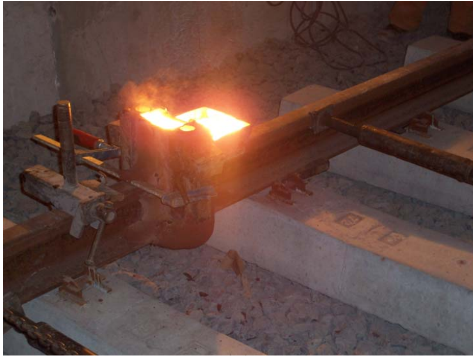
Figure 4.11: Thermite welding application photo taken by Öztürk.E
