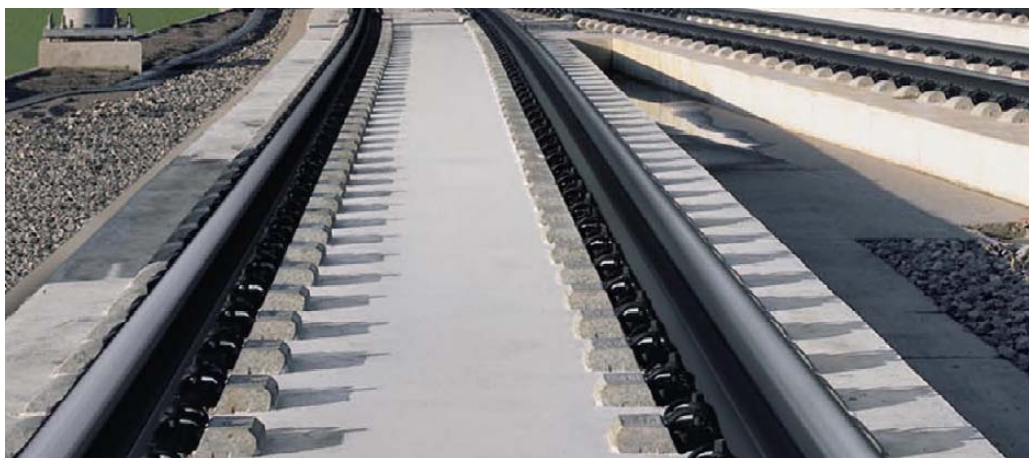
Figure 4.6: Direct fixation track on segregated open area
