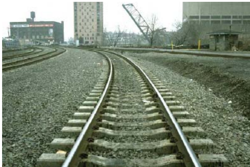
Figure 4.8: Preview of a track with concrete tie
