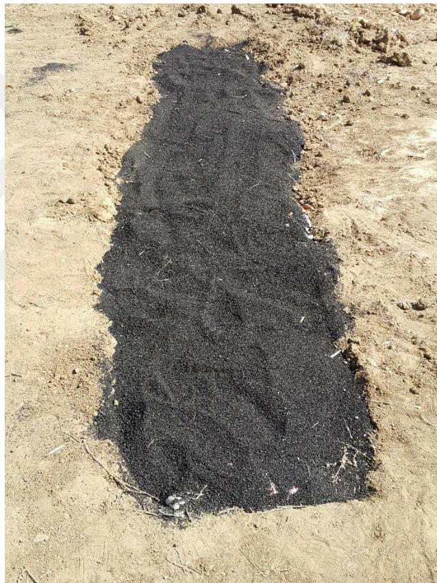
**Figure 3.18. Rubber chip-filled trench**
