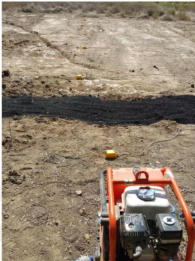
**Figure 3.19. Rubber chip-filled trench setting out**
