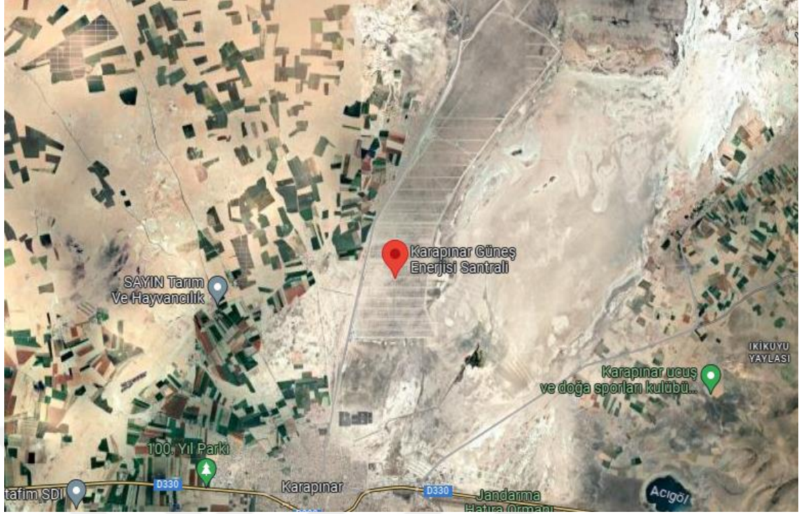
Figure 6.1. Karapınar Solar Power Plant on the map
