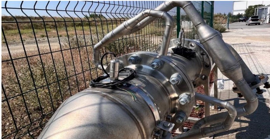
Figure 4-8 Feed line and manifold in setup
