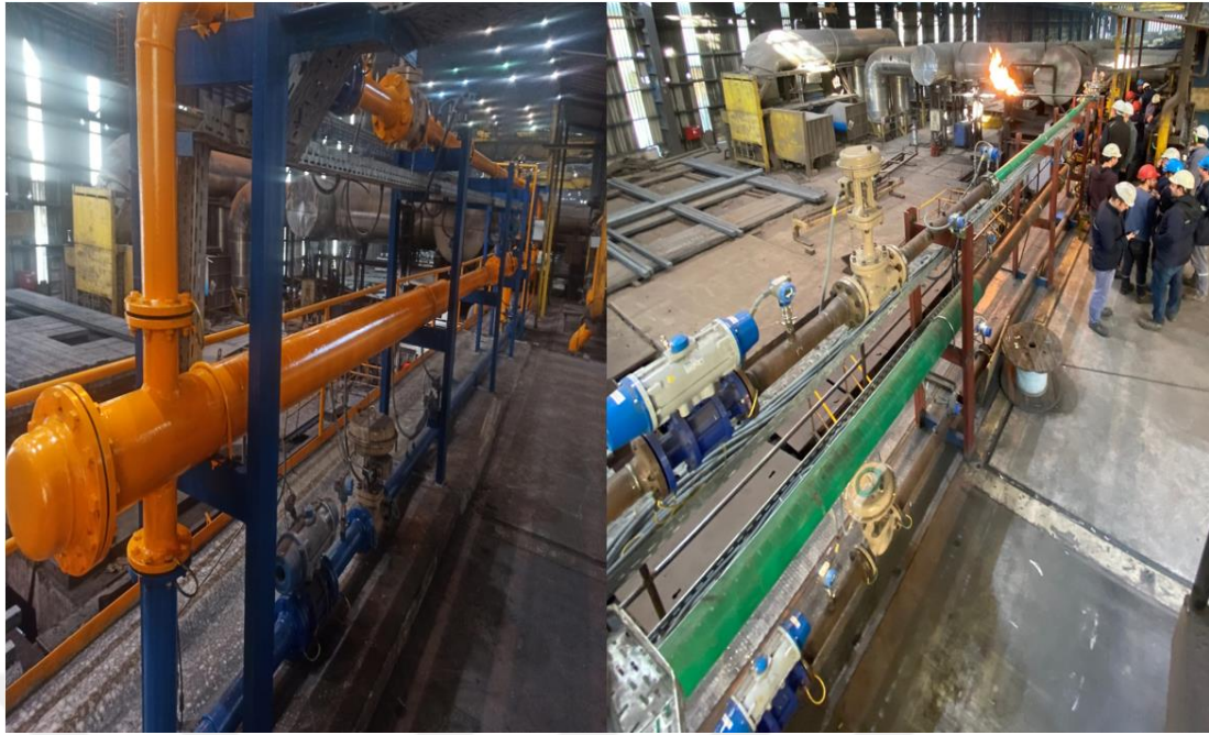
Figure 5.1: LPG-air mixer photos (Used with company permission)
