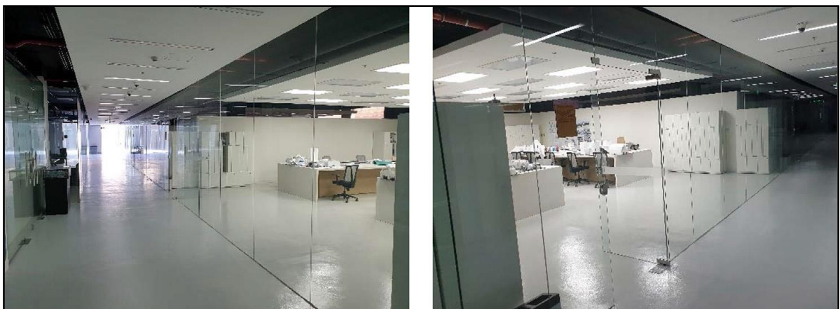
Figure 2.8: Interior Photos for CADD Transition Spaces Display Glazed Partitions on Both Sides of the B and C Spaces that Serve as a Physical and Acoustic Barrier and Maintain Visual Consistency for Classes.
