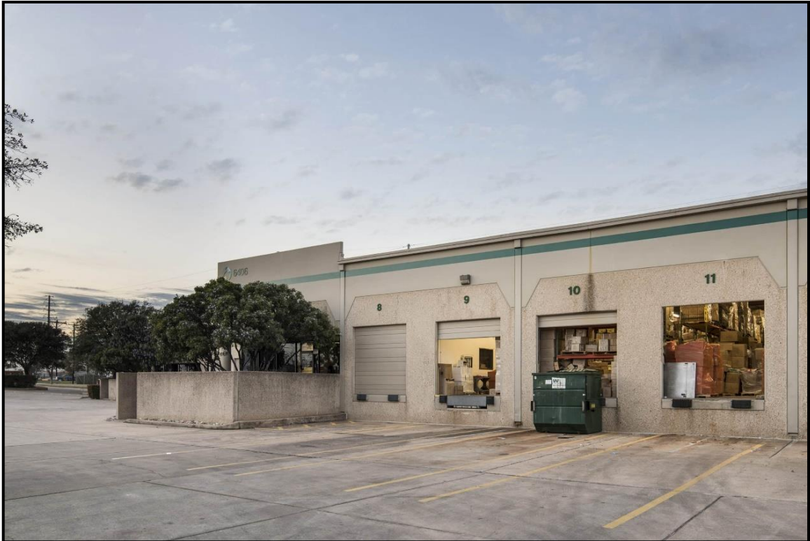
Figure 3.2: High-loading dock doors at the Getagadget Warehouse.
