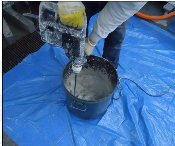
Figure 3.5. Preparation of GGBFS slurry with a stirrer motor.
