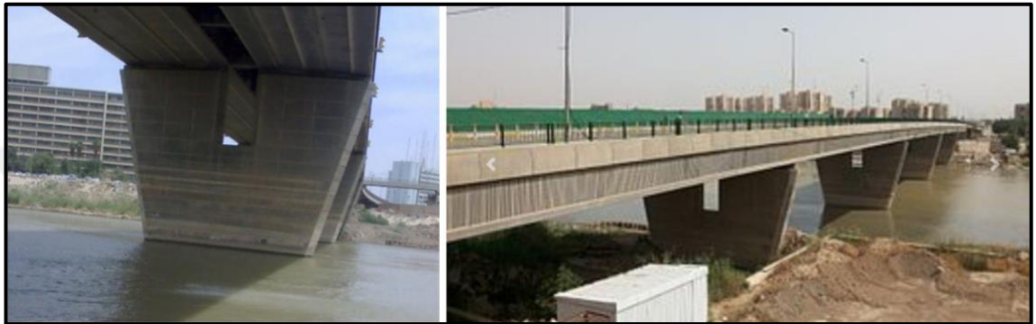
Figure 3.2 The first case study (Bab Al-Muadam bridge)
