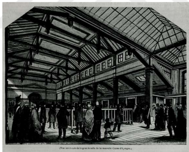
Figure 3.21 : Interior View Of The Great Room Of The New Savings Bank. 20 (L’Illustration, 1845, no. 112).
