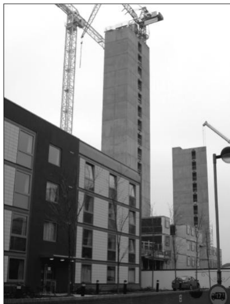
Figure 2.11: Construction of Concrete Cores for a Modular Building (Lawson&Richards, 2010)
