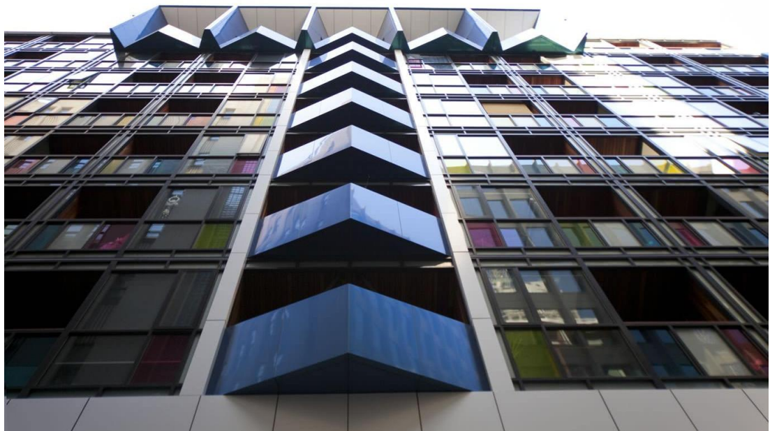
Figure 4.9: Little Hero Building (Fender Katsalidis Australia, n.d.)
