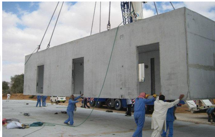
Figure 2.6: Positioning of a Concrete Module with Crane 5
