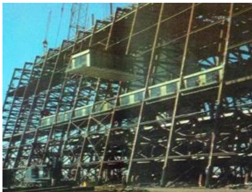
Figure 2.12: Placing a Module into a Framing System (Ramaji&Memari, 2013)
