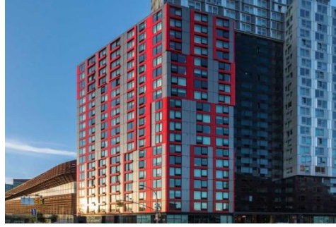
Figure 4.29: B2 Tower (MG McGrath Inc, n.d.)
