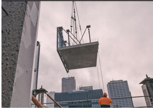
Figure 4.8: Construction of Collins House (Hickory, 2018)
