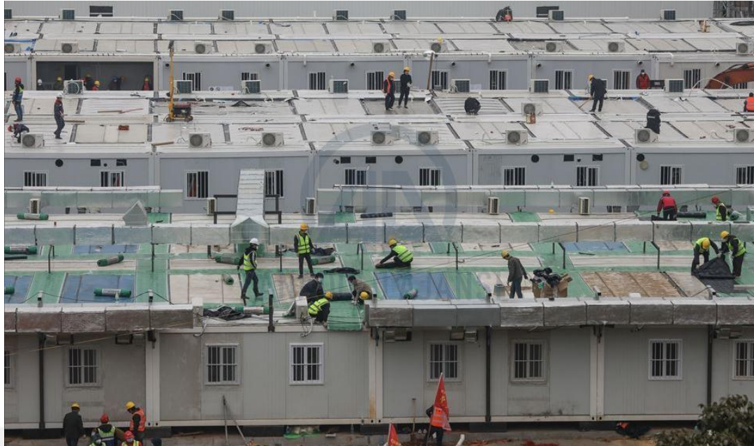
Figure 4.11: Wuhan Huoshenshan Hospital Construction (Stringer – Anadolu Agency, 2020)
