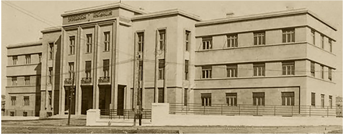
Figure 22. Ministry of Health Building
