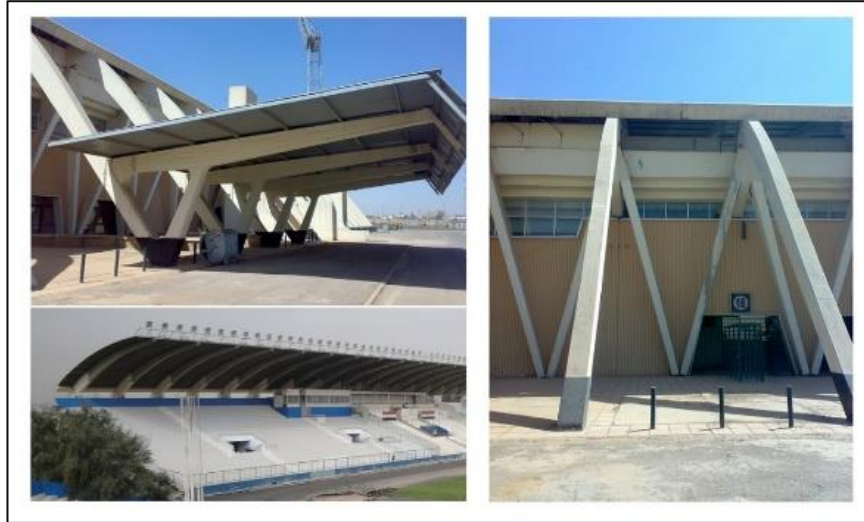
Figure 2. 2 Real photos for the structure of the straight-line stands cover. (Photo by the author Abdullah Allawi)
