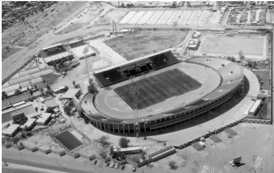
Figure 1. 4 Al-Shaab international stadium [6]
