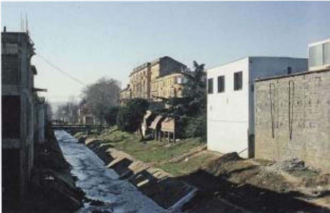
Figure 107: Illegal buildings occupied banks of Lana River.
