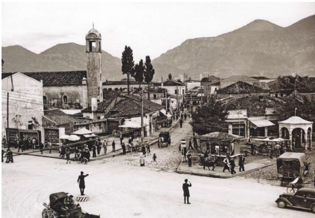
Figure 91: Street Scene (1940) Transition from the modern part of the city to the old part. The new part has wide boulevards with asphalt pavements. Road system is gridiron. The new, modern buildings were usually more than two storey, reinforced concrete, with flat roofs. On the other hand, the old side is full of narrow, stone pavement roads with one or two storey, tile roofed buildings.
