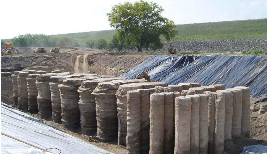
Figure 2.8 Jet Grout columns in the site view
