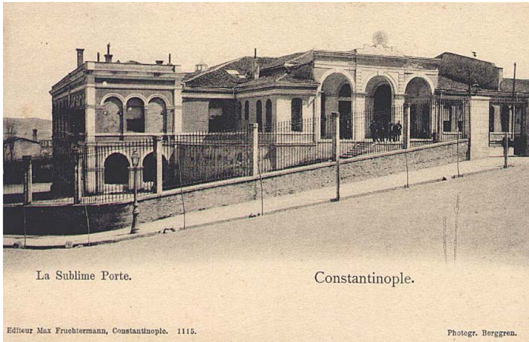
Figure 2.2: The part of the Babiali Building complex towards Cağaloğlu Slope and Babiali Street (Url-2).
