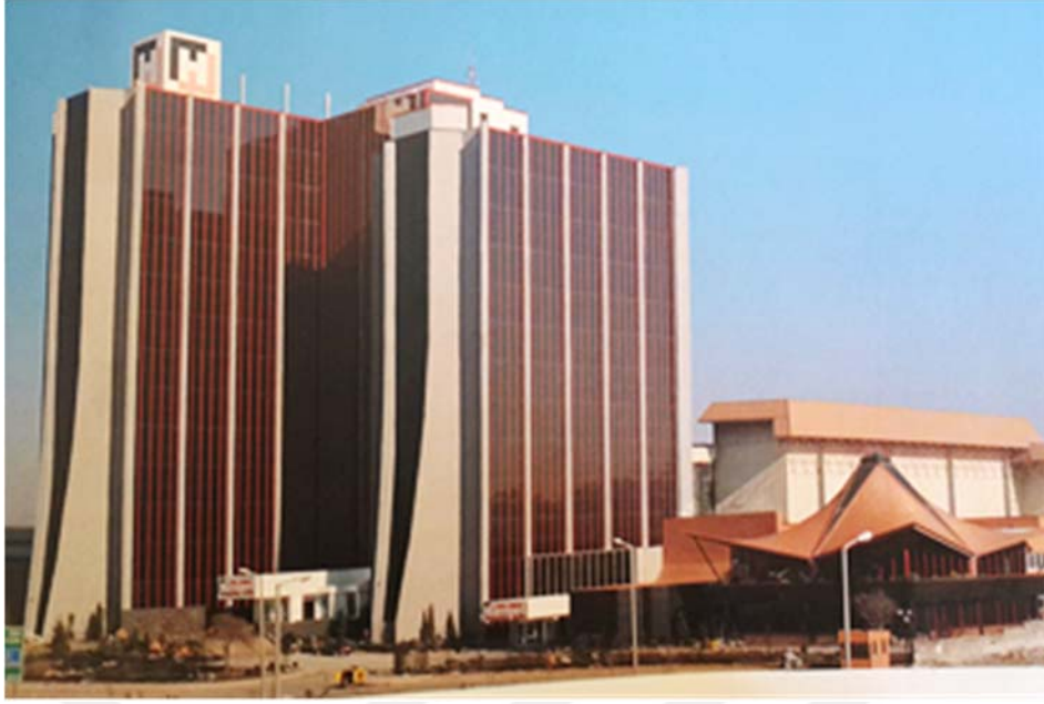
Figure 3.8: An exterior view of Hürriyet Media Towers (Yapı, 1994).
