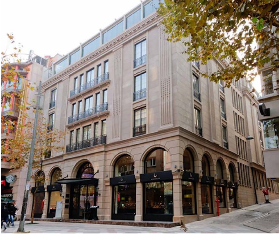
Figure 2.12: The remodelled exterior of the building (Url-7).
