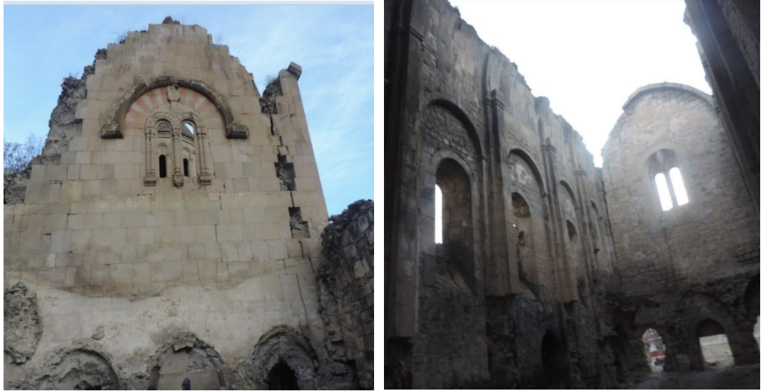
Figure 4.8: The Crack on the Western Facade of the Church and the Completely Collapsed Roof Section.
