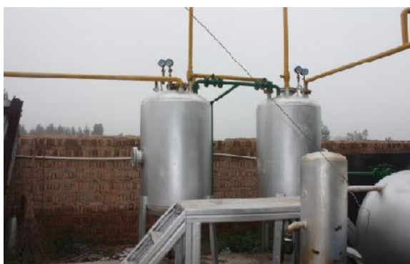
Figure 3.18. Water seal.
