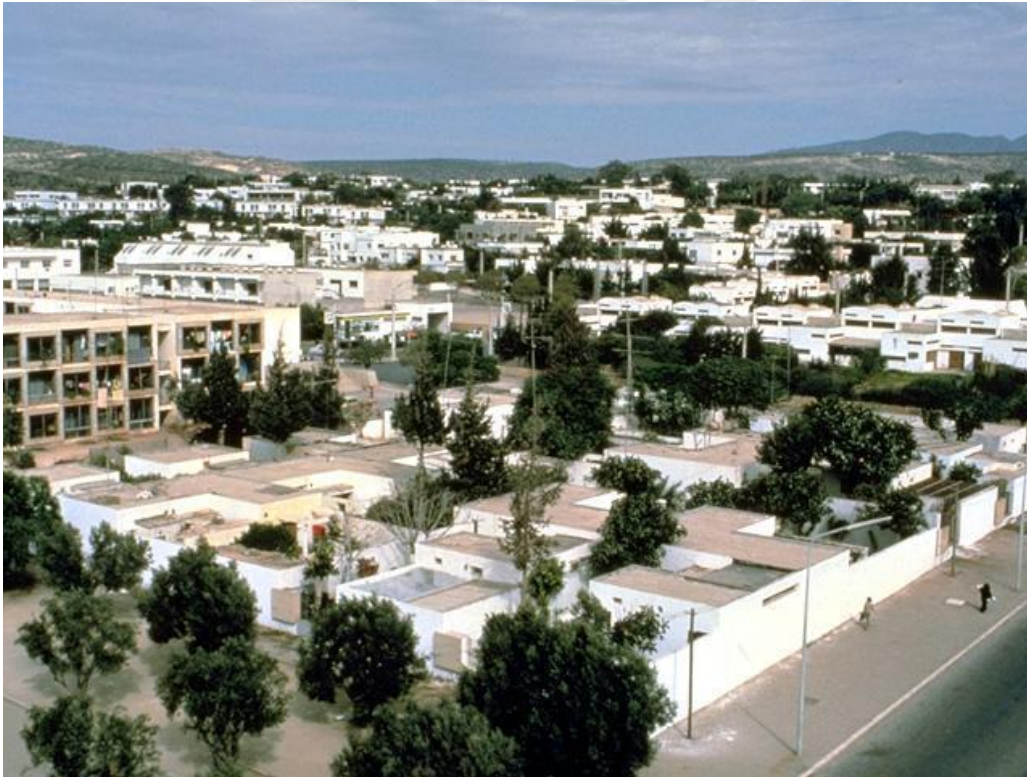
Figure 3.8. Aerial view of the Courtyard Houses, Agadir, Morocco
