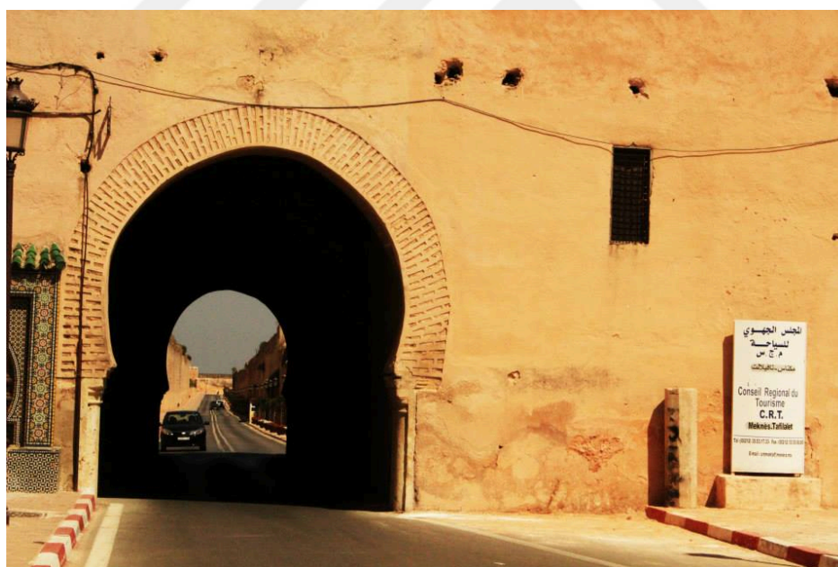
Figure 2.17. The surrounding walls of the city in Meknes.
