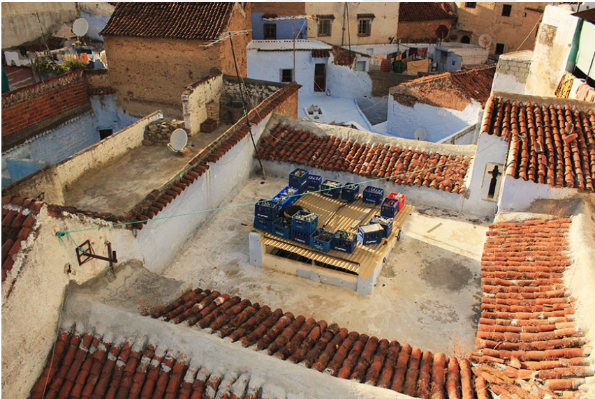
Figure 2.6. A photograph from the top of a house, Chefchaouen, Morocco, where the daylight from the roof is passed to the courtyard of the house.
