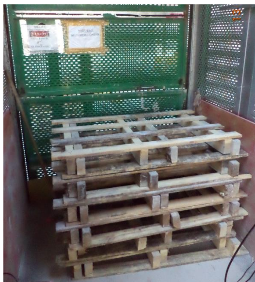
Figure 4.5 : Empty pallets loaded on the elevator and removed from the floor.
