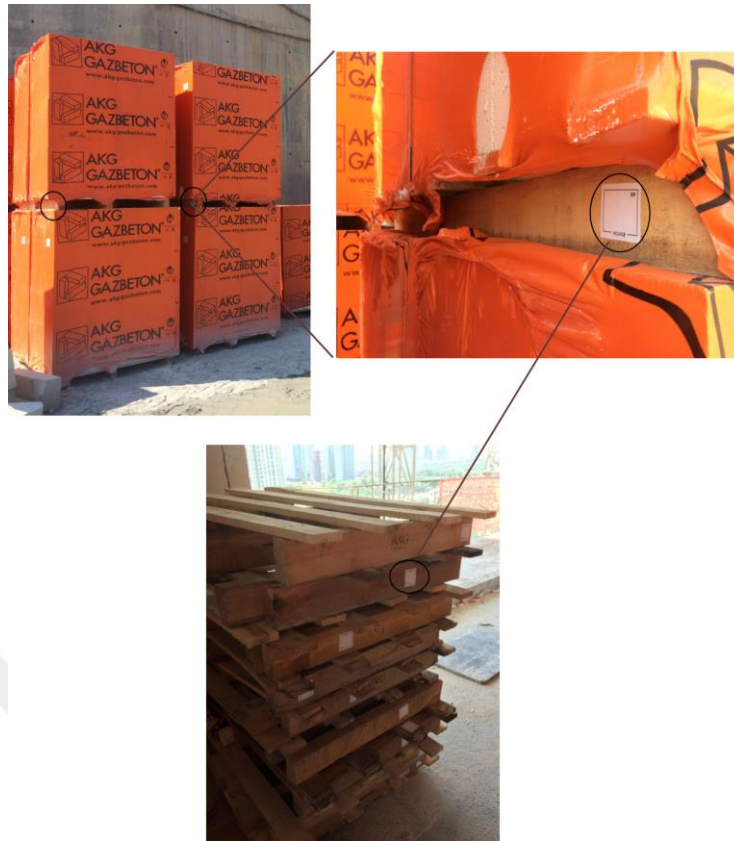
Figure 4.10 : RFID tags on AAC pallets before the unwrapping of packaging, and after the AAC blocks are utilized and pallets are emptied.
