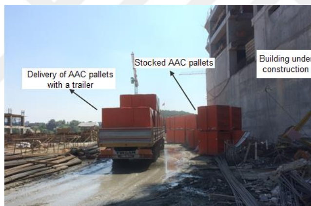
Figure 4.2 : A trailer delivering the AAC pallets to site.
