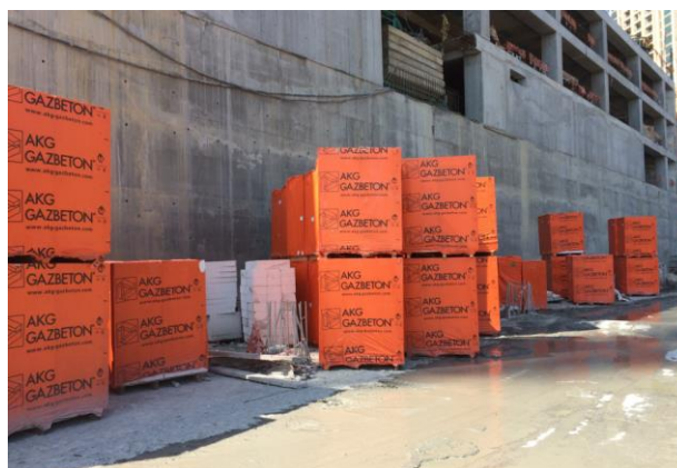
Figure 4.3 : AAC pallets stocked at the laydown area.
