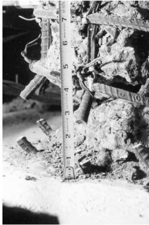
Figure 3.44 : Hines et al. (2002) – Test unit 1A fractured longitudinal bars at the end of the test.
