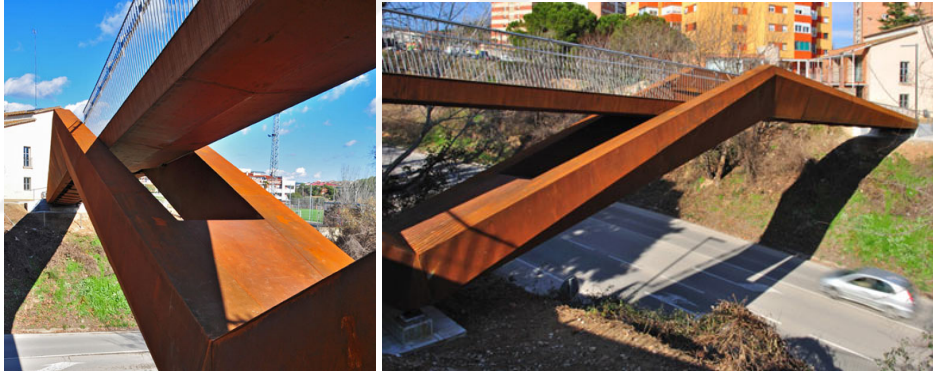
Şekil 2. 20 Can Gili Footbridge (Spain, 2009) [37]
