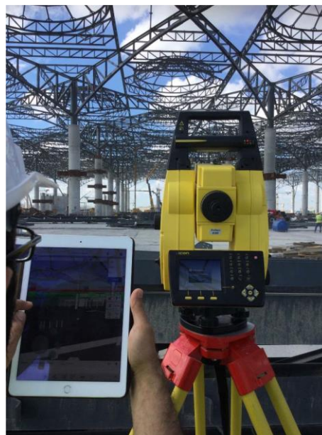
Figure 3.20 : Controlling site installation with BIM360 Layout application.
