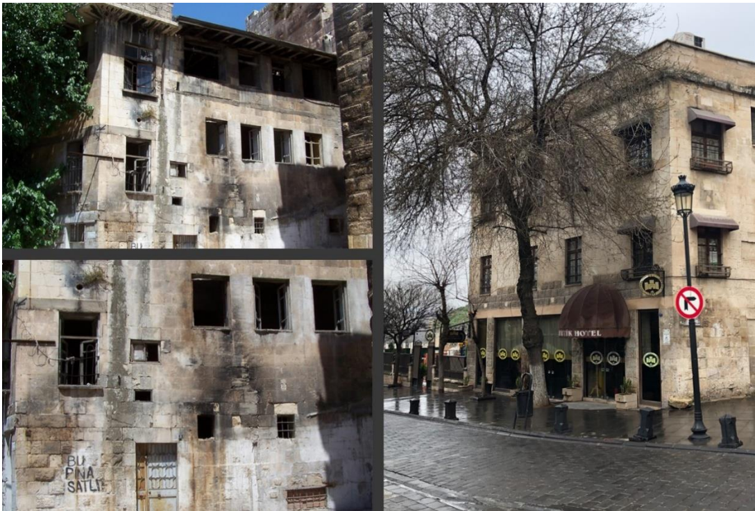
Figure 4.26. Renovation of Boutique Hotel (Source: Kutay İnşaat, 2019)
