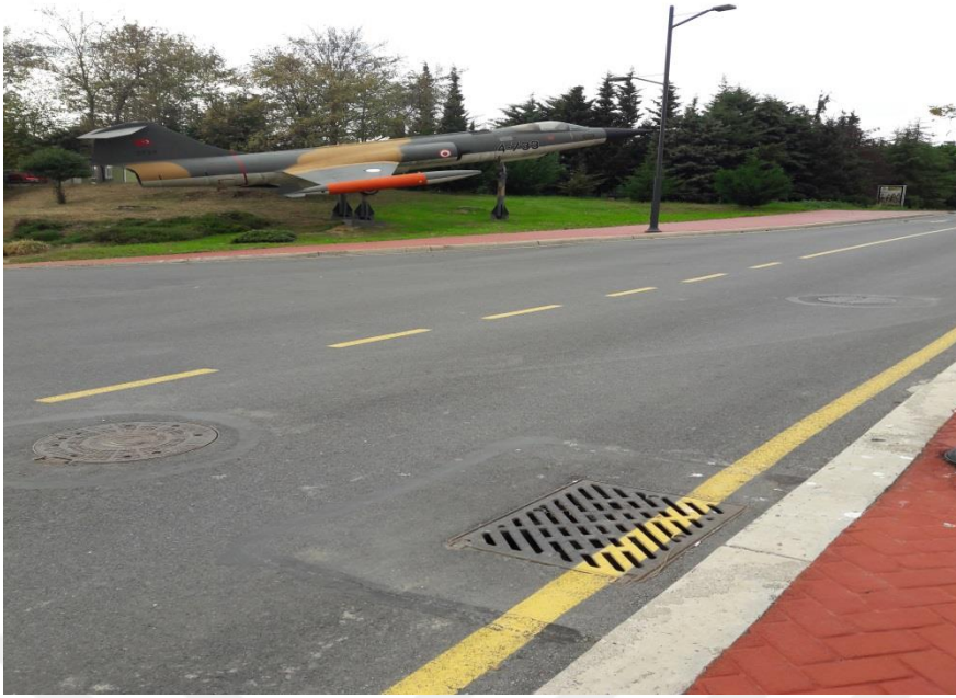
Figure 2.7: One sample of rain water inlet point at ITU main campus.
