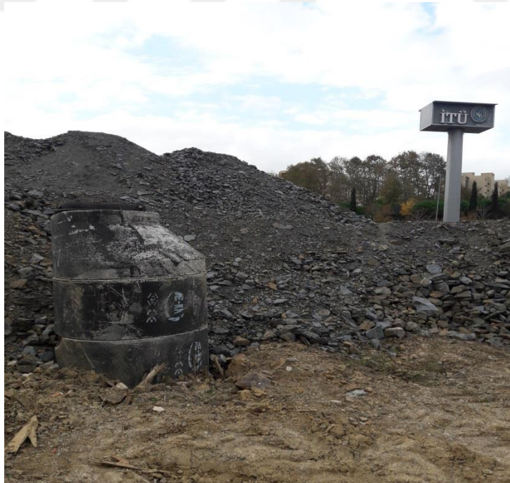
Figure 2.8: Main outfall point of the ITU main campus drainage system.
