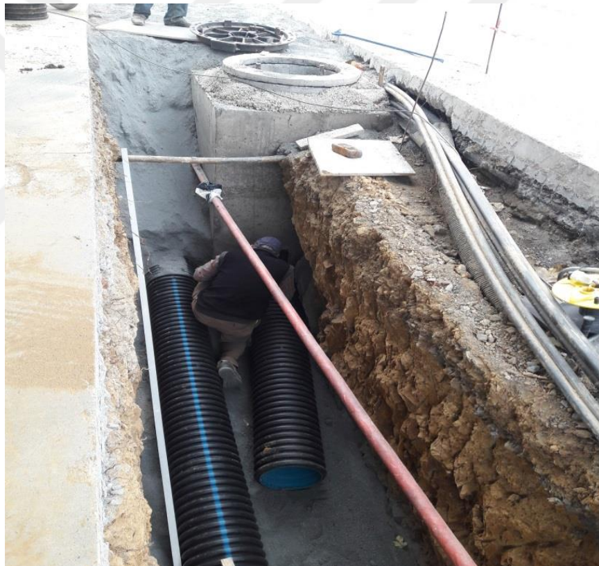
Figure 2.6: Drainage & Sewer pipe lines, ITU Main Campus.
