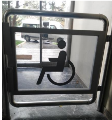
Figure 4.52. Entrance for wheelchair users
