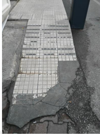
Figure 4.29. Narrow and deformed curb ramp
