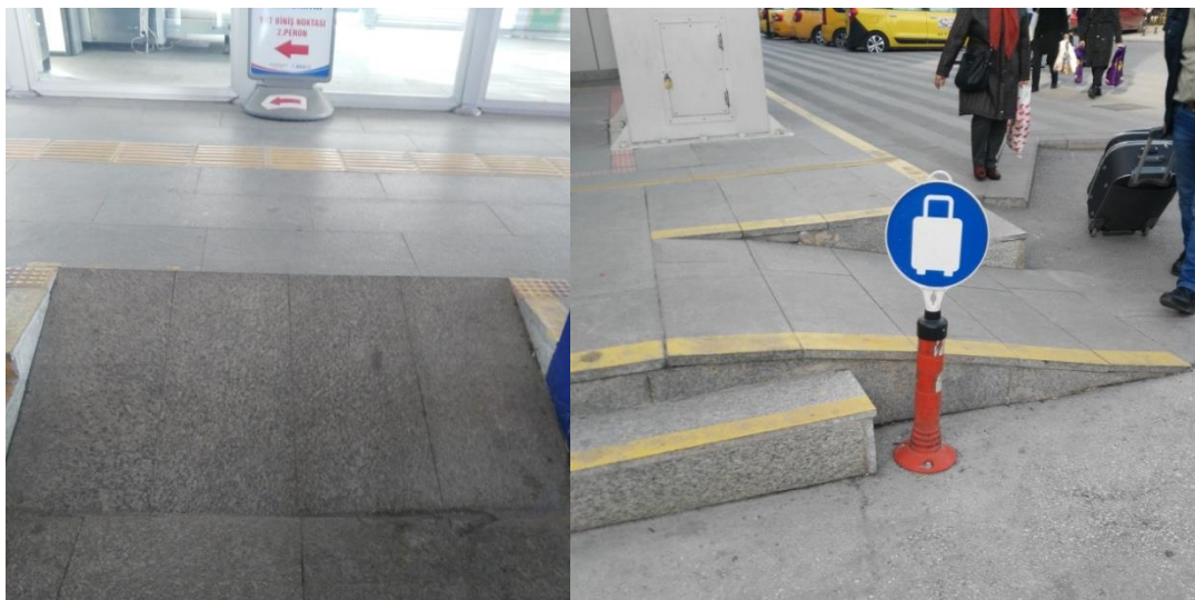
Figure 4.11. Vertical ramps not having tactile walking surfaces
