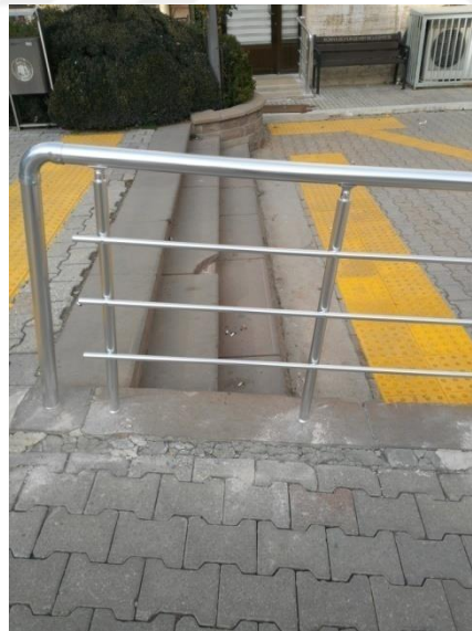
Figure 4.43. Stairs with tactile surface and handrail
