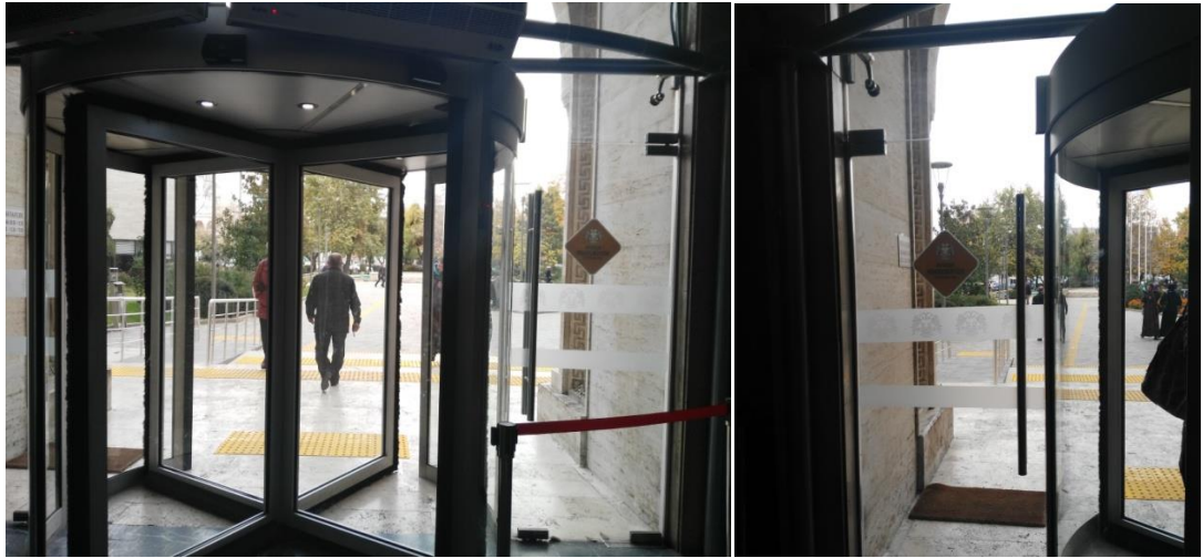
Figure 4.50. Revolving door and hinged door at entrance
