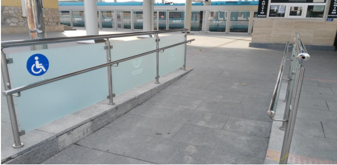
Figure 4.6. A ramp for wheelchair users
