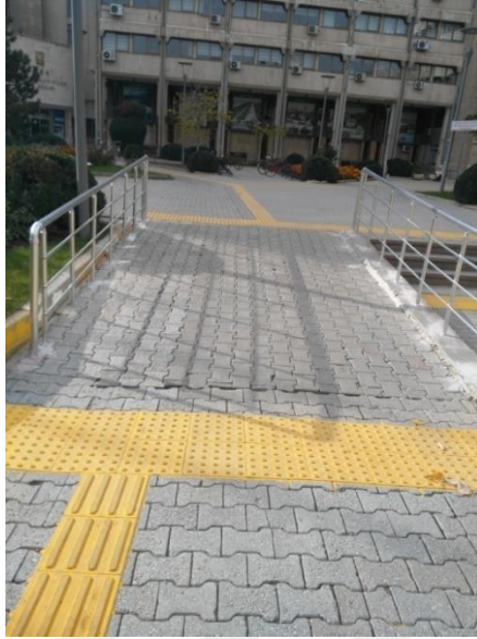
Figure 4.42. Tactile walking surfaces at exterior environment
