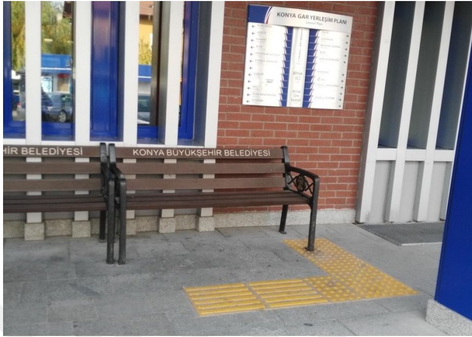
Figure 4.7. A discontinuous and non-functional tactile walking surface
