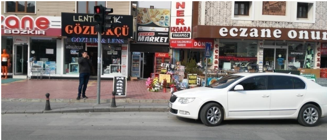
Figure 4.20. Discontinuity of curb ramps on pedestrian crosswalk
