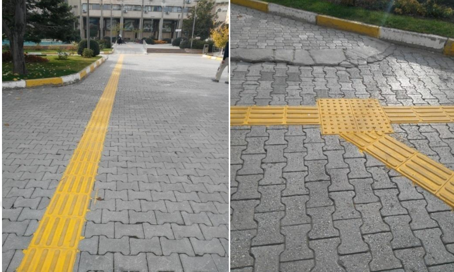
Figure 4.44. Tactile surfaces at outside of the municipality
