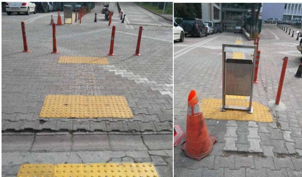
Figure 4.22. Tactile surfaces occupied by different materials
