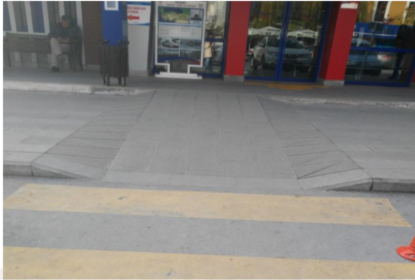
Figure 4.4. A curb ramp intersecting pedestrian crosswalk
