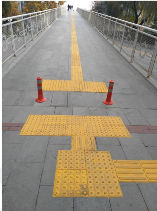
Figure 4.41. An overpass through metropolitan municipality
