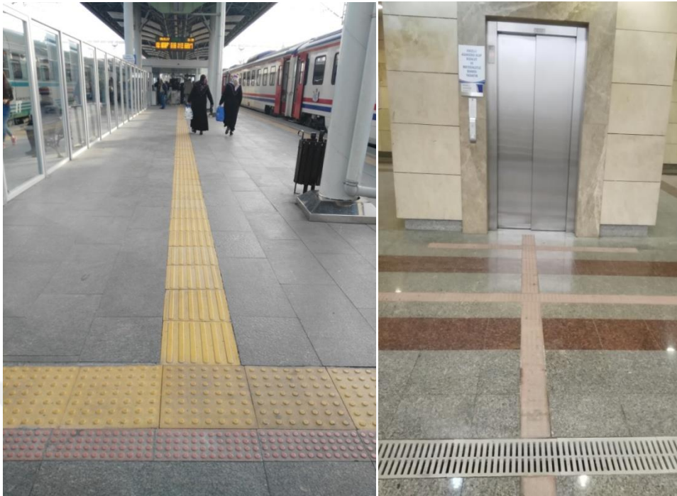
Figure 4.13. Tactile walking surfaces inside of the railway station
