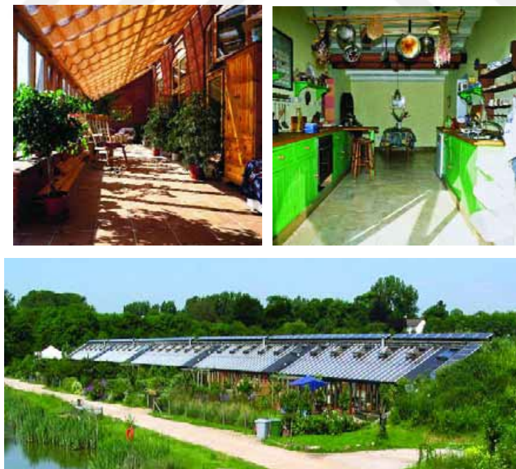
Figure 3.34: 1) The south-facing conservatory acts as a large suntrap. 2) The slab construction is left exposed internally in this room, allowing the walls and ceilings to contribute thermal mass. The tiled floor provides Additional thermal mass, which creates a thermal link to the ground floor slab. 3) Exterior view of Hockerton Housing Development (Walsh et al., 2006)
