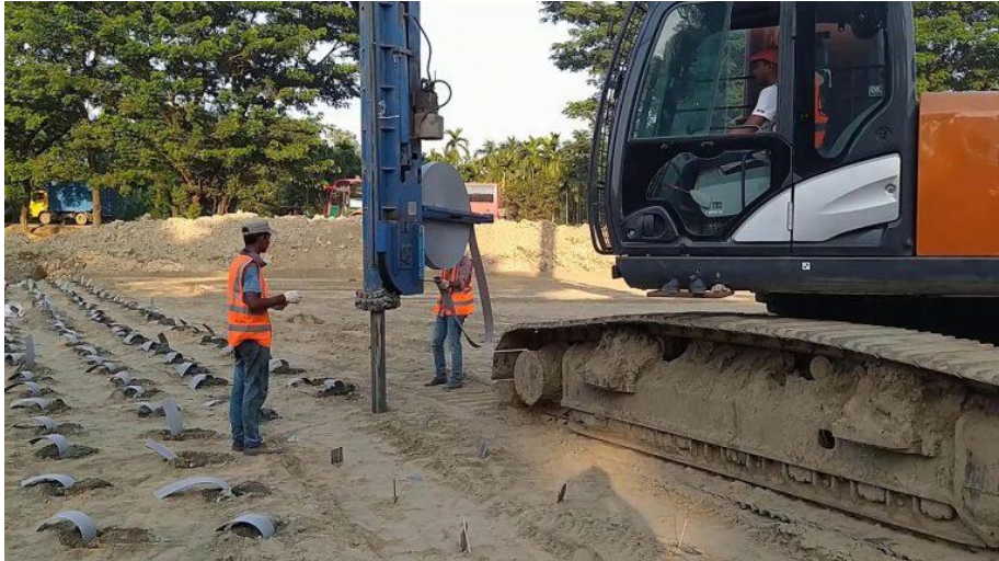
Figure 2.4. Mandrel-installed Prefabricated Vertical Drains at a site https://gssb.com.my/sand-drain-vs-wick-drain-what-difference
