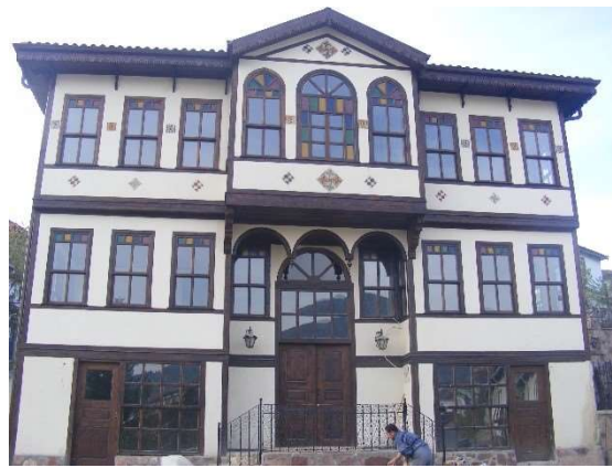
Figure 4.23. Post-intervention view of east side facade (Author, 2013)
