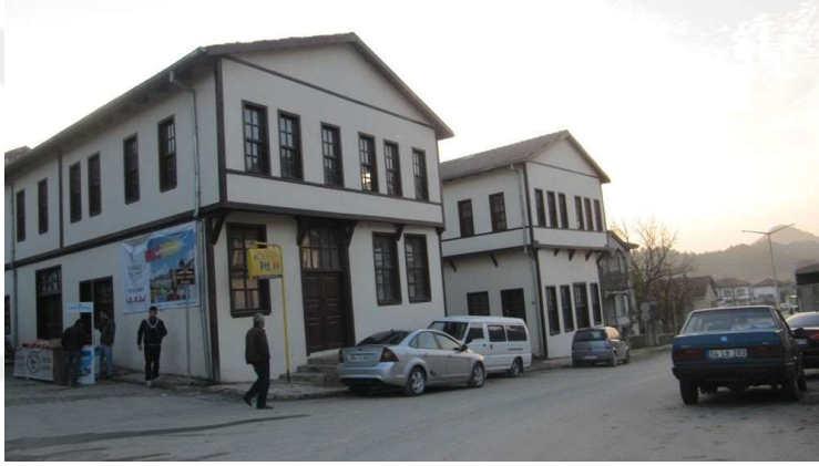
Figure 2.7. Hacı Hatun Han after its restoration (Author, 2013)
