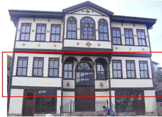
Figure 4.8. A1. Post-intervention view of east side facade that show the alterations of windows at first floor (Author, 2013)
