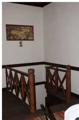
Figure 3.48. Post-intervention view of staircase, FPOI08 (Author, 2016)
