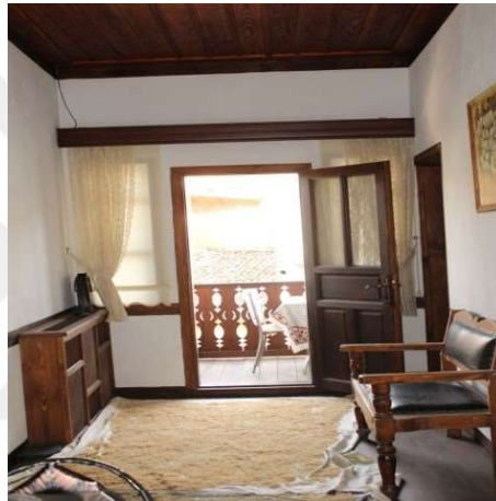
Figure 3.47. Post-intervention view of hall, FPOI08 (Author, 2016)
