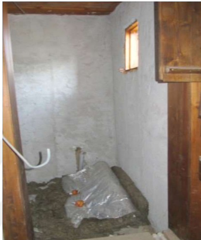
Figure 3.70. Wet space addition inside the closets at rooms of mezzanine floor (Author, 2013)
