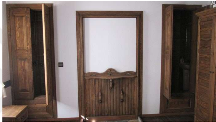
Figure 4.35. G.A1, closets that were altered and transformed into bathroom and wc in GPOI07 (Author, 2013)
