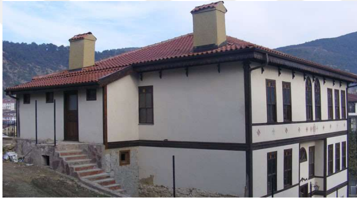
Figure 4.29. Post-intervention view of west facade (Author, 2013)
