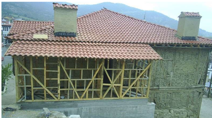
Figure 4.30. Pre-intervention view of west facade (Author, 2013)
