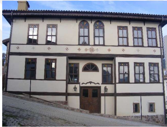
Figure 4.32. Post-intervention view of south facade (Author, 2013)
