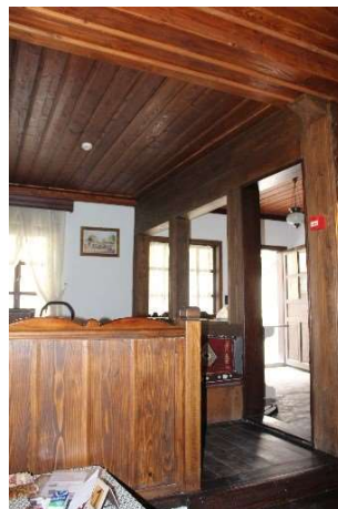
Figure 4.39. Post-intervention views of GPOI08 (Author, 2013)
