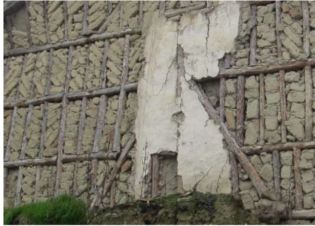
Figure 2.13. Mudbrick detail as a construction material from unnamed house in Taraklı (Author, 2016)
