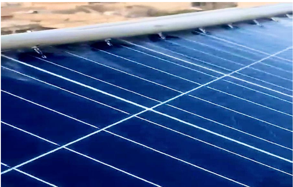
Figure 4.3 Install the nozzle on the surface of the solar panel.
