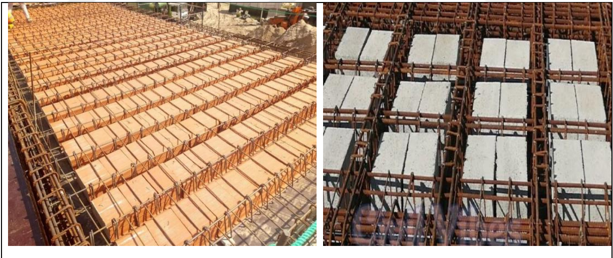
Figure 1.1: An architecture of (a) one-way ribbed slab [19], and (b) two-way ribbed slab [20].
