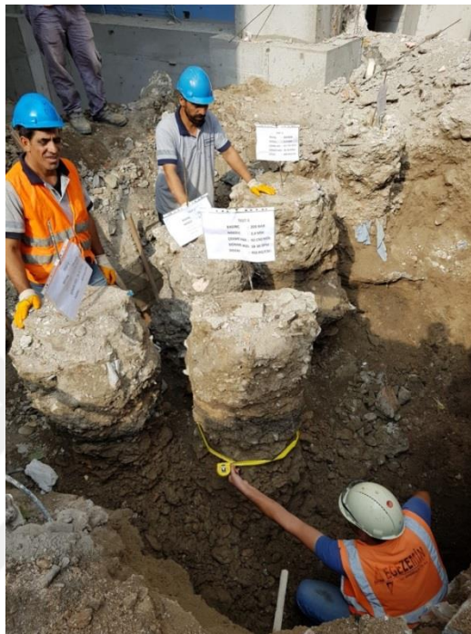
Figure 3.17. Discrete jetgrout columns.
