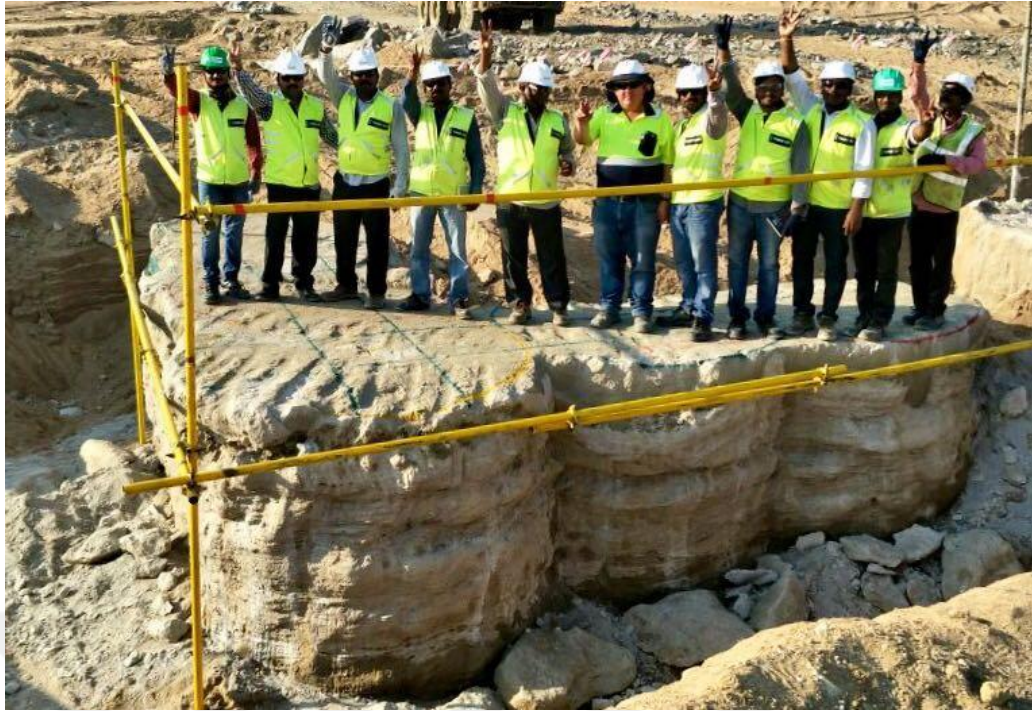
Figure 3.21. Test columns (Source: Kellerindia.)
