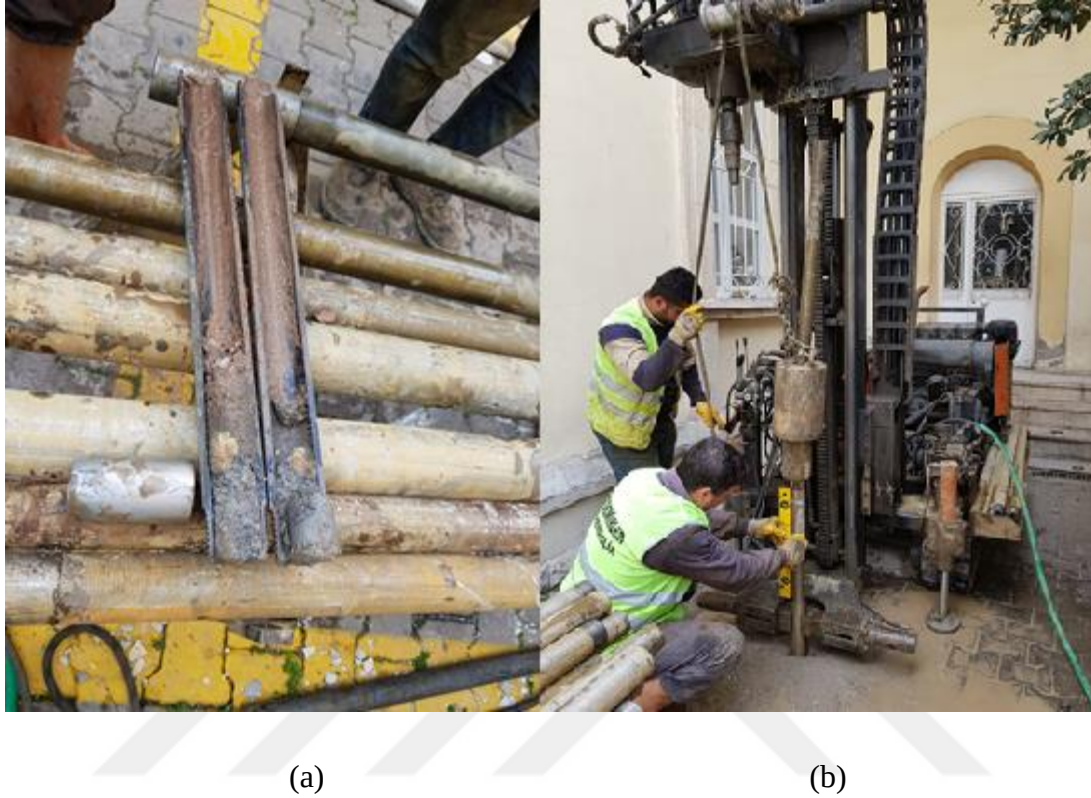
Figure 4.5. SPT sampler (a) and testing (b).
