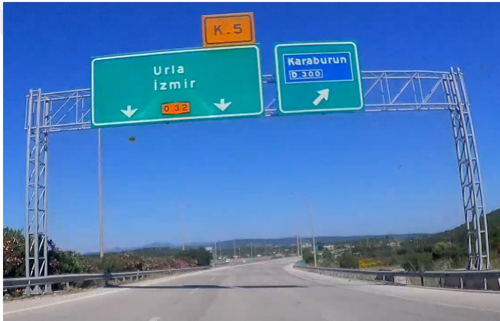
Figure 7. Motorway overhead directional information signs
