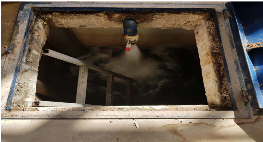
Figure 4.7 Main Water Tank (Reservoir)
