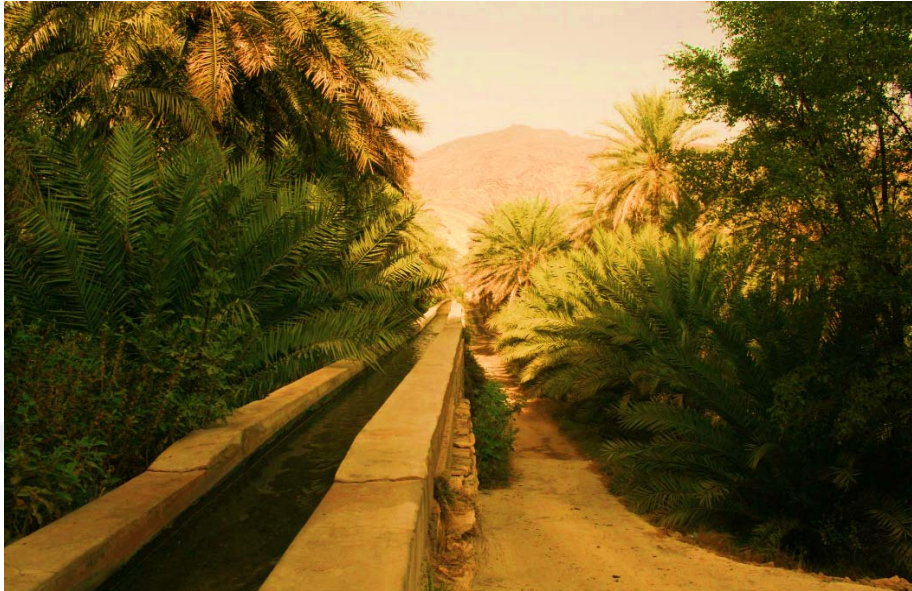
Figure 2. 2. Irrigation canal supplied with water by a qanat or falaj in Oman (Niemann, 2007)
