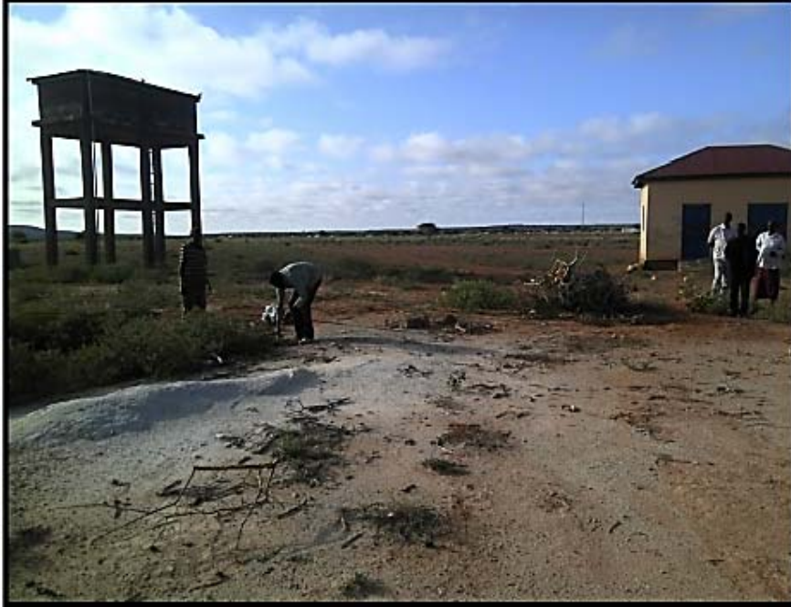
Figure 5. 17. Qoryale town abandoned borehole with Water scheme construction (SHAAC. 2014).
