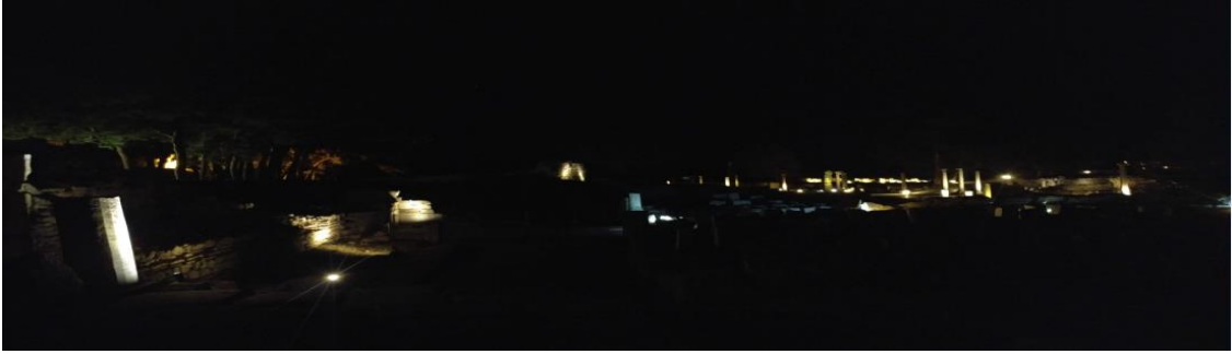
Figure III.13 Ancient City of Ephesus, Izmir. Lighting
