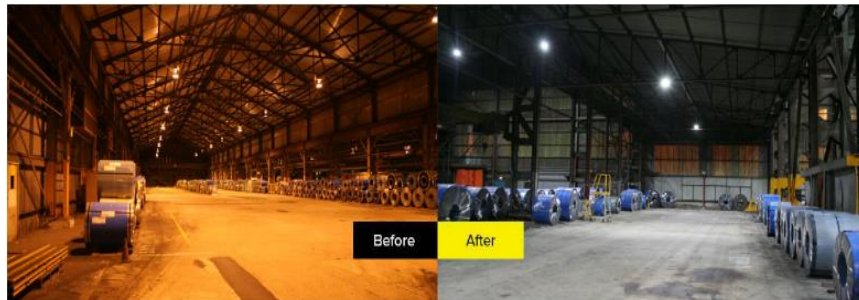
Figure II.5 Difference Between Sodium Vapor Lamp and Color Rendering Values of LED Luminaires [9].
