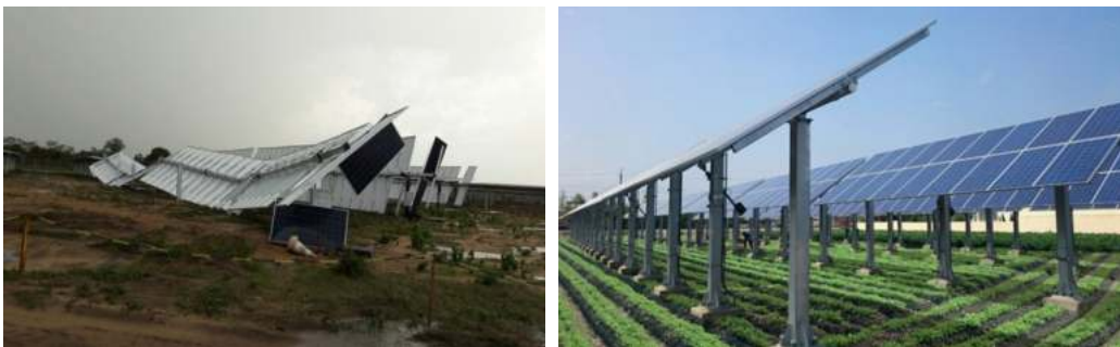
Figure 1.5 Example of PV tracker array and photo of a wind damaged system
