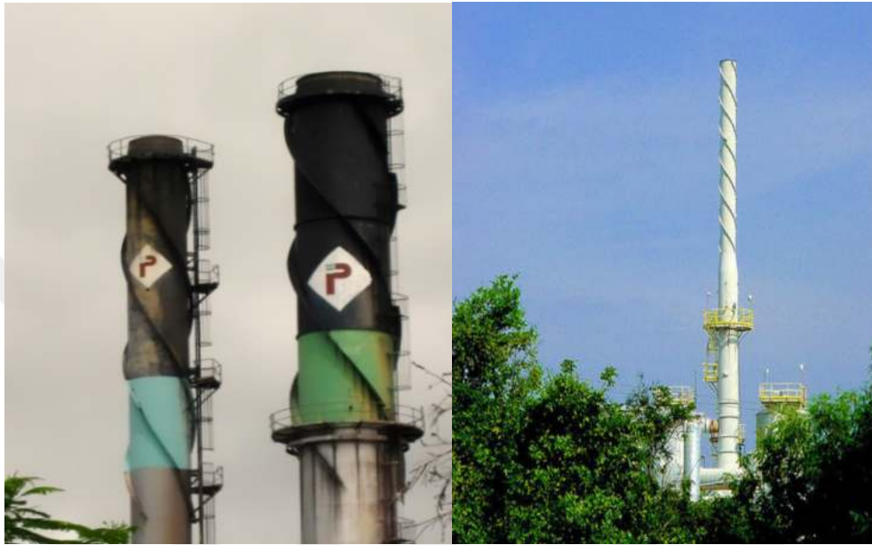
Figure 2.11 Helical wrapping to prevent vortex shedding
