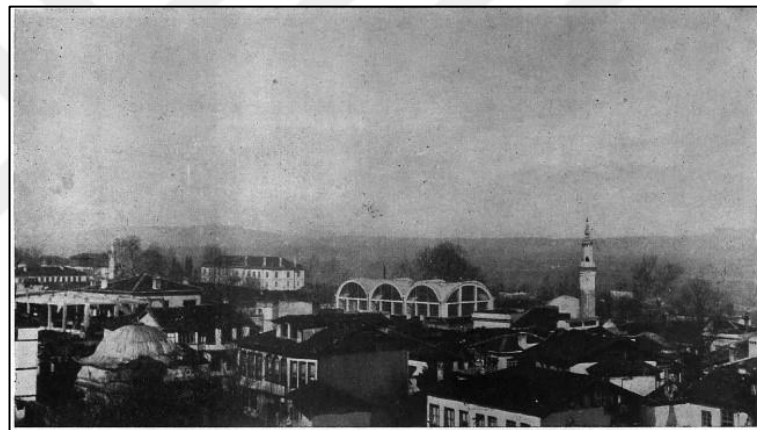
Figure 3.22: A view of Marketplace Building (Femir & Akozan, 1950)
