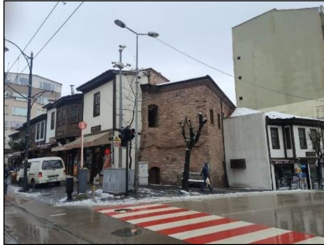
Figure 4.30: Galle Khan after renovation (Bursa Metropolitan Municipality)
