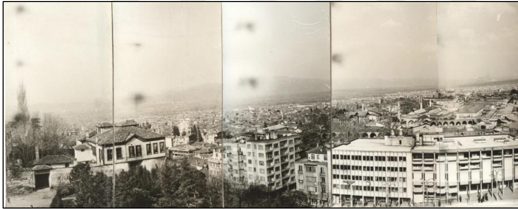
Figure 4.23: General view of urban fabric from Bursa, Tophane in the 1970s (Bursa Metropolitan Municipality Archive)
