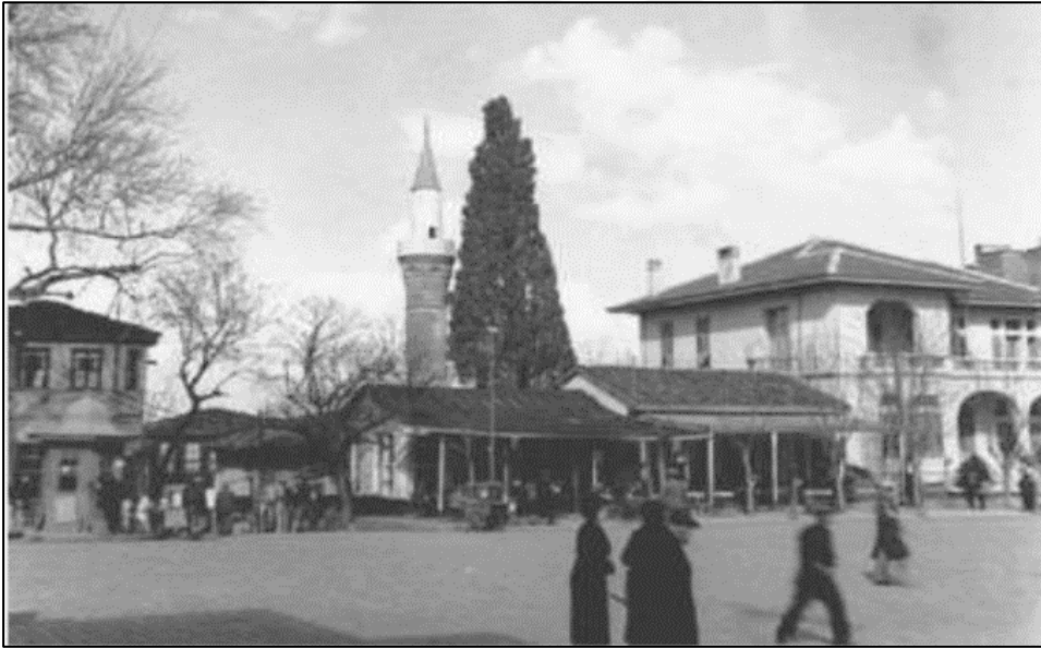
Figure 3.41: Alaca Masjid and CHP building in 1937 (Url-25)
