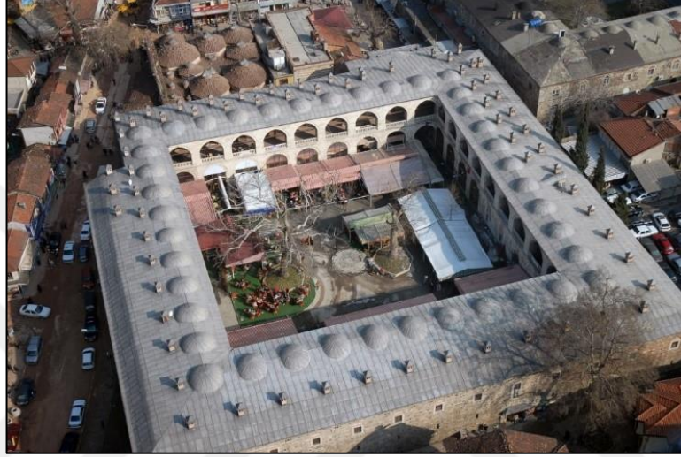
Figure 4.31: General view of Pirinç Khan, after restoration project (Url-38)
