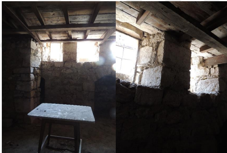
Figure 2.26 South wall in the basement floor (Şahin Güçhan, 2019)
