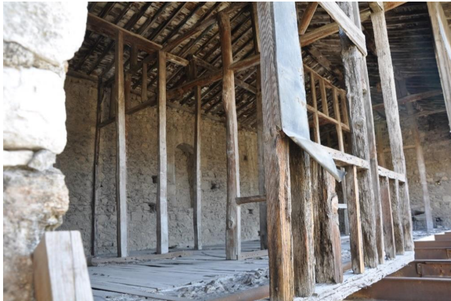
Figure 2.41 First floor timber frame (METU CONS, 2019)
