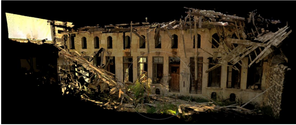
Figure 2.47 Point cloud created by 3D laser scanning (METU TAÇDAM, 2023)
