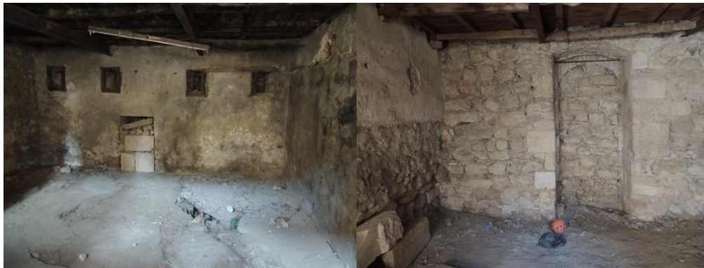
Figure 2.20 Filled door openings in B01 and B03 (Şahin Güçhan, 2019)
