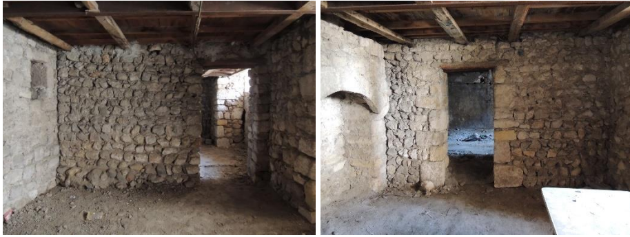
Figure 2.30 Partition walls in the basement (Şahin Güçhan, 2019)
