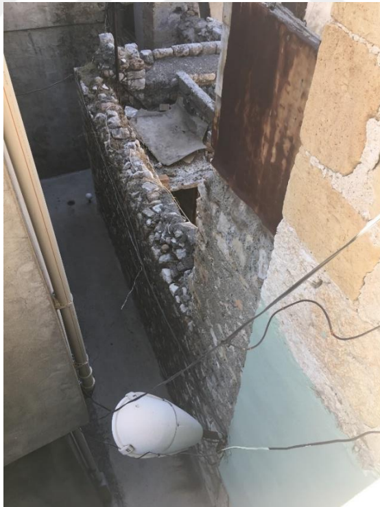
Figure 2.28 East wall and courtyard wall (Şahin Güçhan, 2019)
