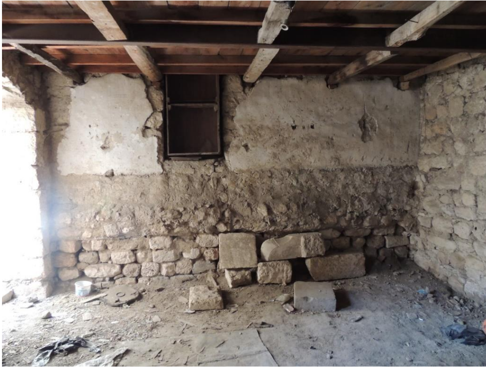
Figure 2.22 Basement west wall (Şahin Güçhan, 2019)
