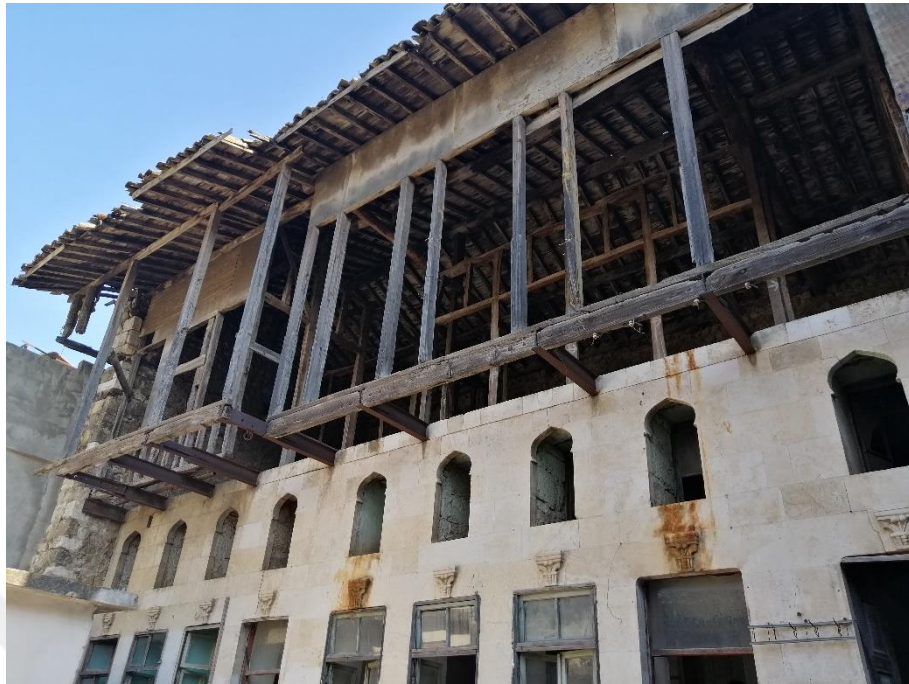
Figure 2.44 Unfinished facade of the first floor (METU CONS, 2019)
